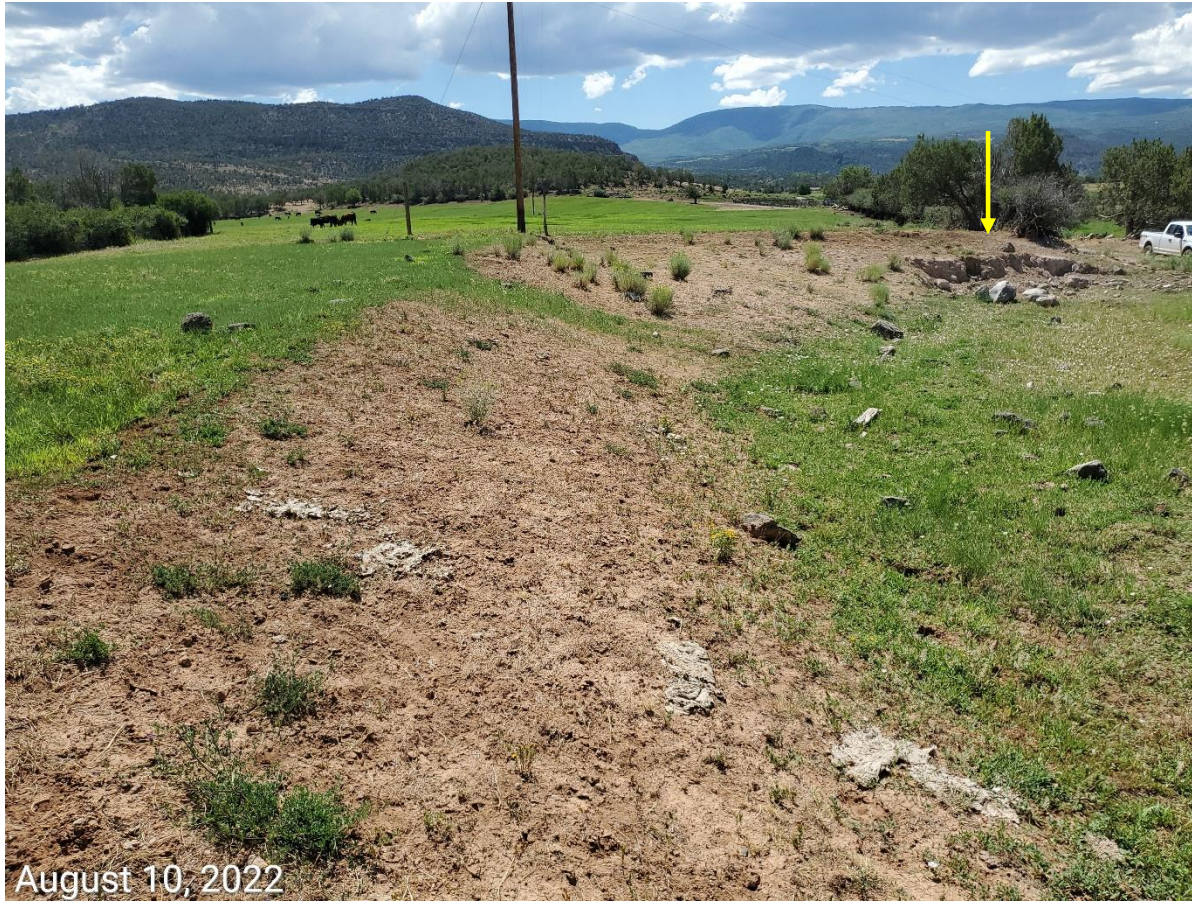
Photo 5: Photo shows cut slopes remaining on the Locaiton. Photo also show areas observed in photo 3 where erosion degradation has persisted.
