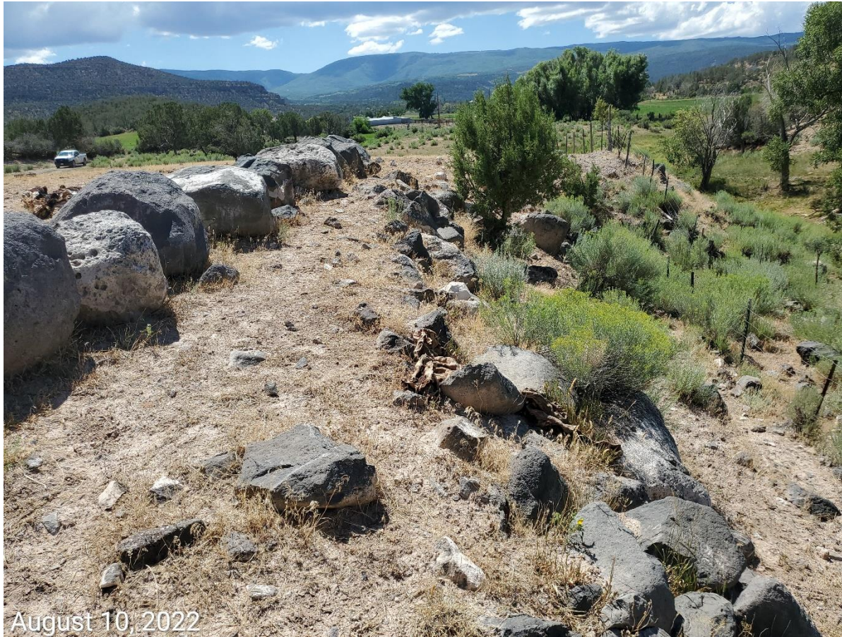
Photo 6: Photo shows fill slopes remaining on the Location.
