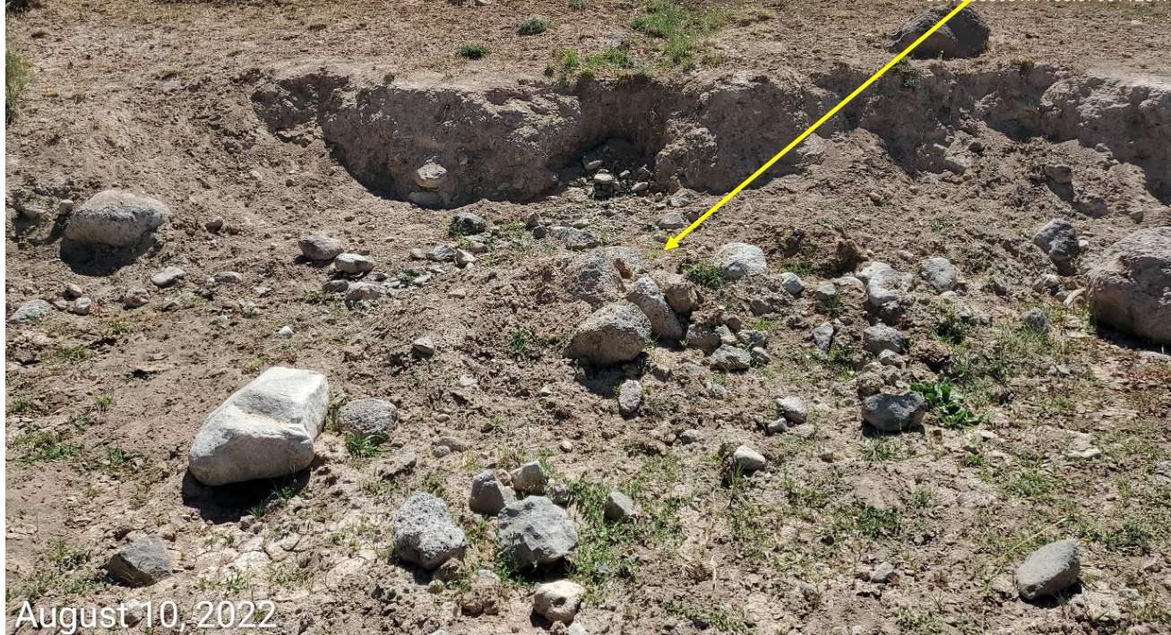
Photo 3: Photo taken from the cut slopes. Photos in the top left/right of the corner taken from the 7/7/2021 inspection. Photo center shows cut slopes have continued to erode. Stormwater BMPs remain missing/insufficient.
