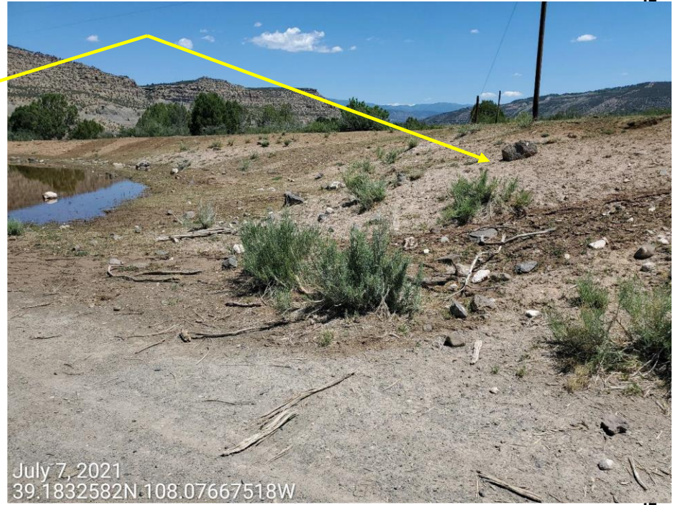
Photo 4: Continued from photo 3. Photo right from the 7/7/2021 inspection. Photos a comparison showing the degradation of the cut slope.
