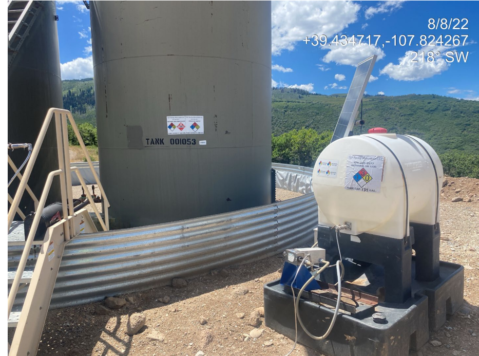
Photo 3. Photo shows methanol tank has been labeled, addressing a previous corrective action.
