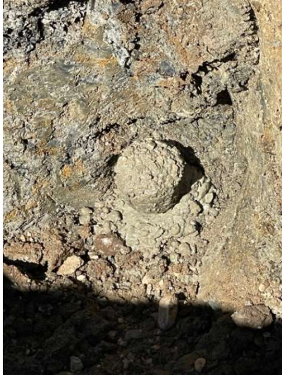
Riser excavated, cut, cement capped, and covered.
