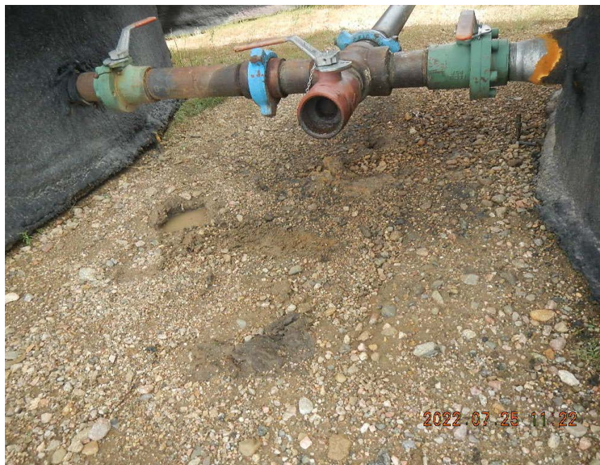
Tank 0030, staining beneath hammer unions. Possible weeping of fluids from valve.
