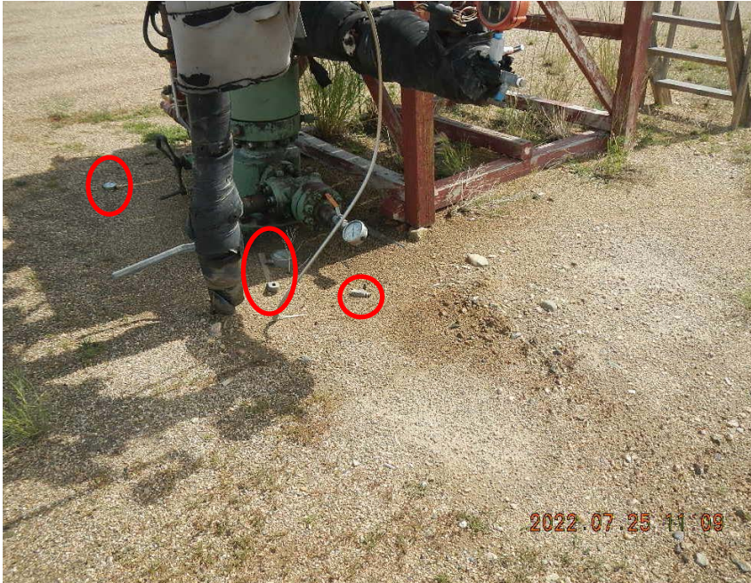
Staining from May 2021 gas leak/vent and condensate around wellhead. Trash/unused equipment (wrenches, needle valve and pressure gauge).
