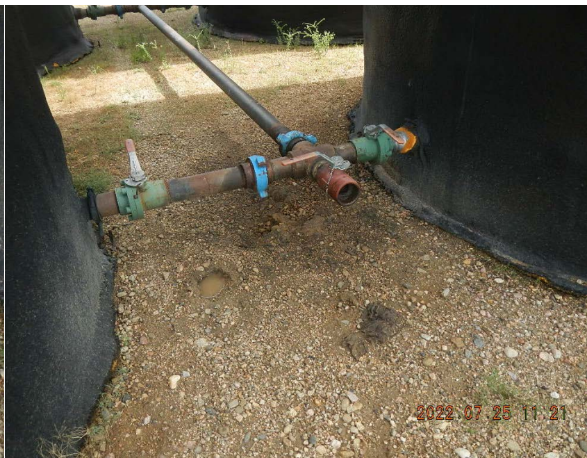
Tank 0030, staining beneath hammer unions.
