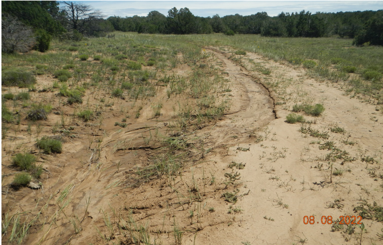
Photo 3. Facing southeast further along the access road. There is additional erosion along the road that has occurred from a recent storm event. Previous corrective action for additional stabilization of the road was not completed.
