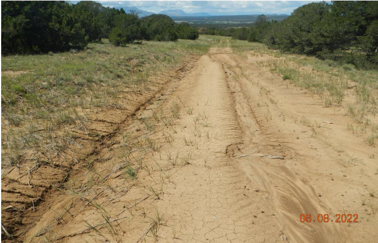
Photo 4. Facing northwest further along the access road. There is additional erosion along the road that has occurred from a recent storm event. Previous corrective action for additional stabilization of the road was not completed.
