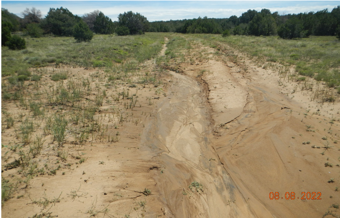
Photo 2. The road then turns back to the southeast. There is additional erosion along the road that has occurred from a recent storm event. Previous corrective action for additional stabilization of the road was not completed.
