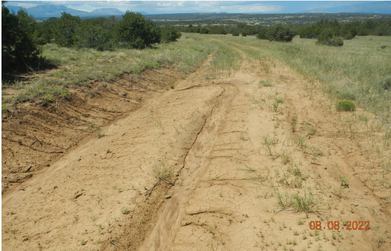
Photo 5. Facing south east further along the access road. There is additional erosion along the road that has occurred from a recent storm event. Previous corrective action for additional stabilization of the road was not completed.
