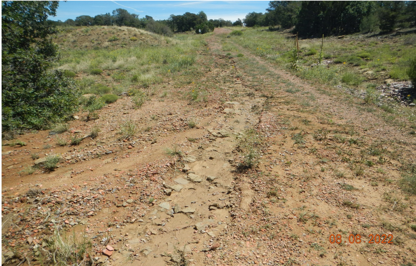
Photo 1. Facing southeast along the access road. There is erosion occurring along the road that has not been repaired and has worsened since previous inspection. Previous corrective action not completed
