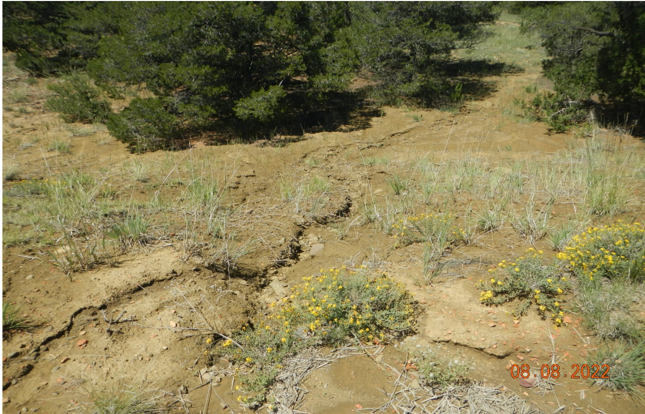
Photo 5. Facing toward the fill slope. There erosion occurring along the fill slope which is not stabilized.
