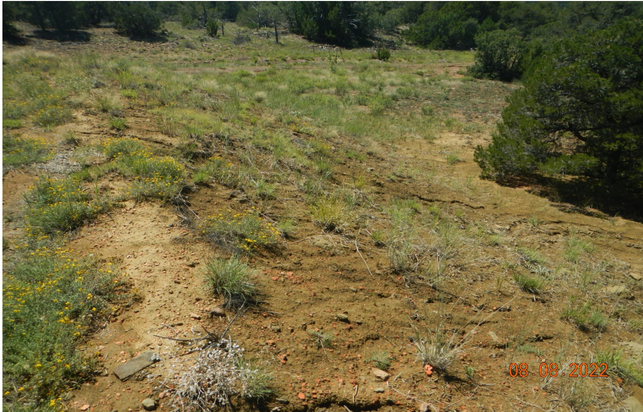
Photo 4. Facing toward the fill slope. There erosion occurring along the fill slope which is not stabilized.
