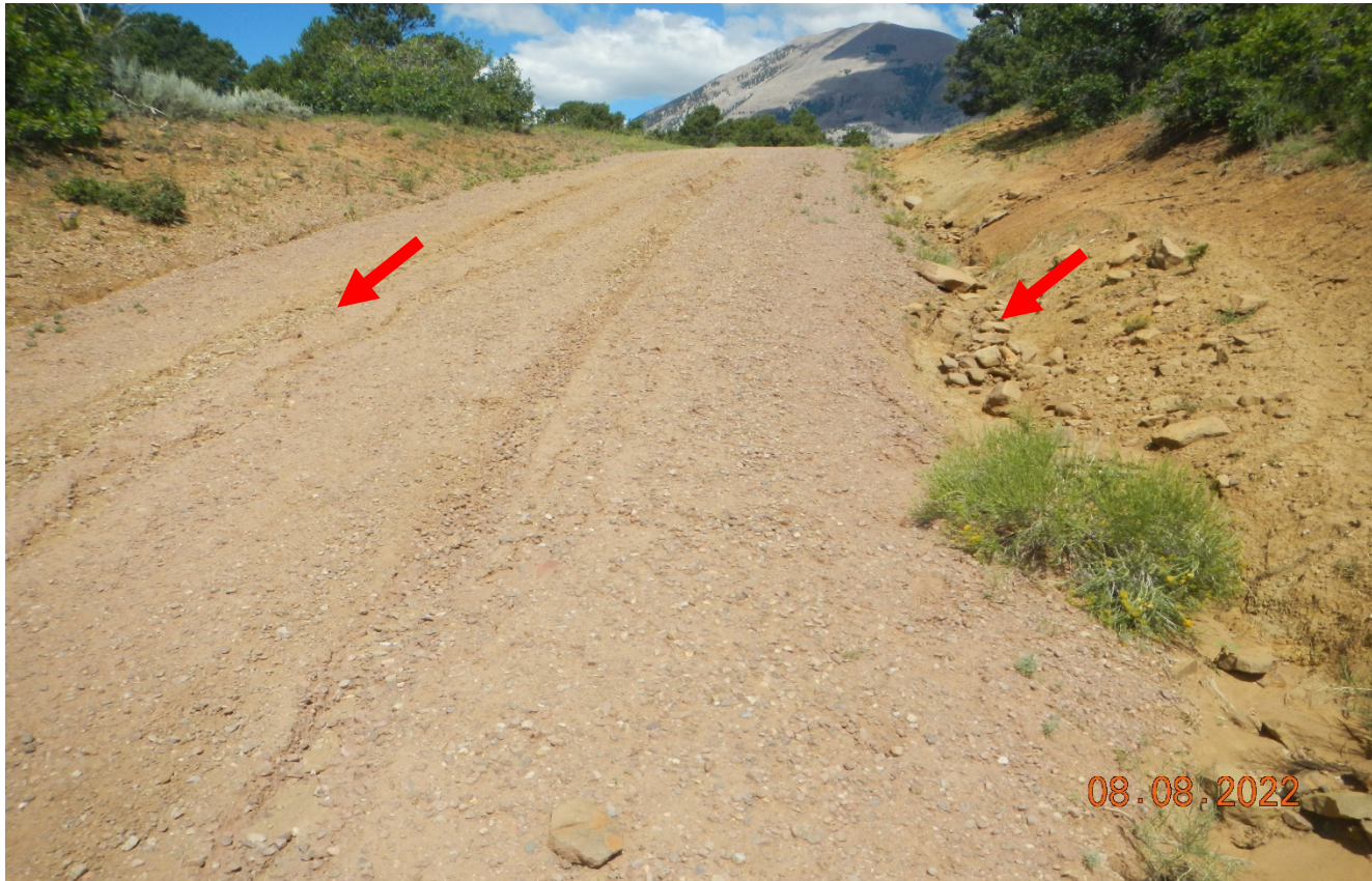
Photo 4. Facing northwest along the road. There is erosion along the road that needs to be repaired and stabilized.
