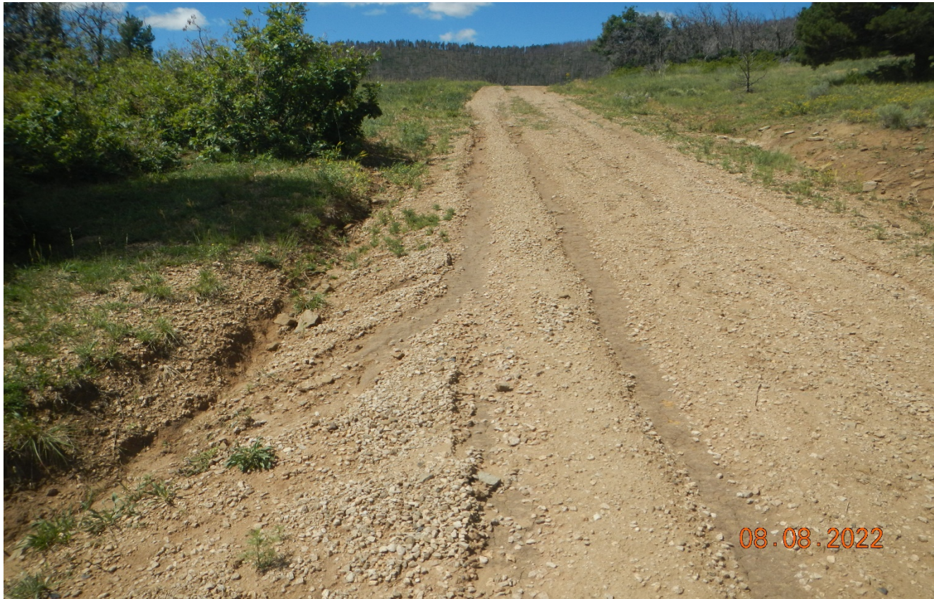
Photo 6. Facing southwest along the road. There is erosion along the road that needs to be repaired and stabilized.
