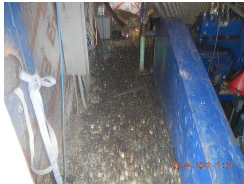
Oil stained ground and gravel inside of pump house.
