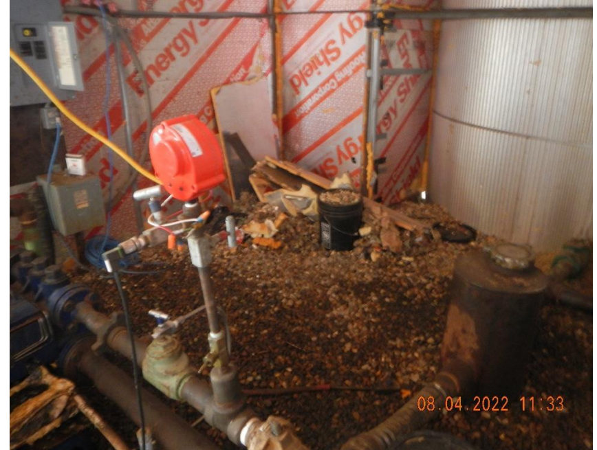
Oil stained ground and gravel inside of pump house. No secondary containment.
