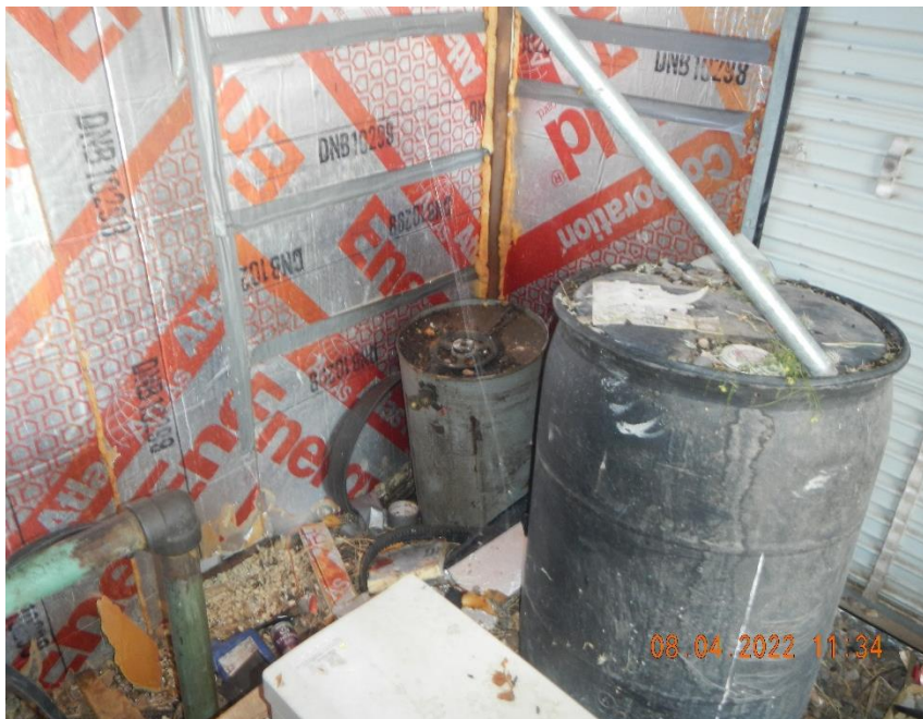
No secondary containment for stored drum and bucket.
