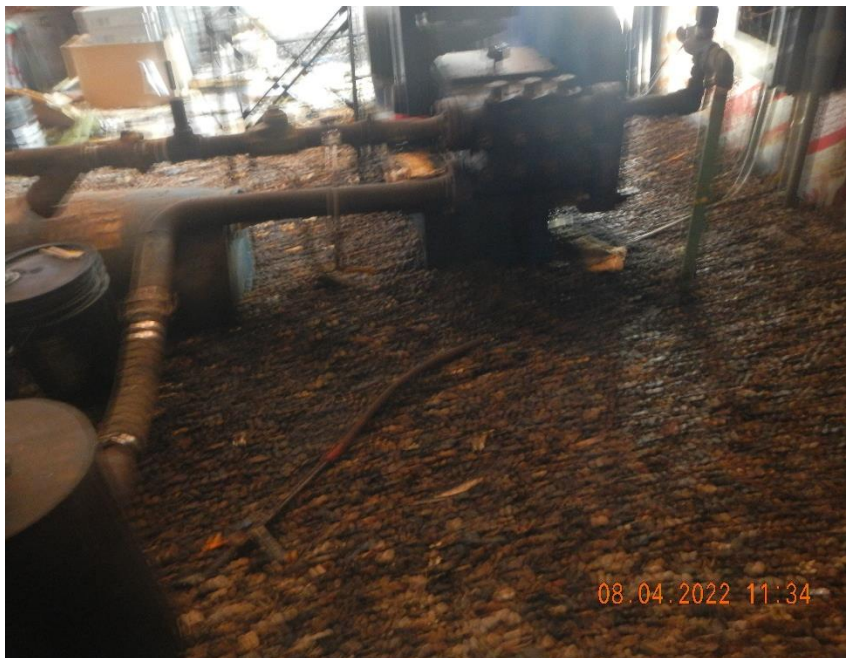
Oil stained ground and gravel inside of pump house. No secondary containment.
