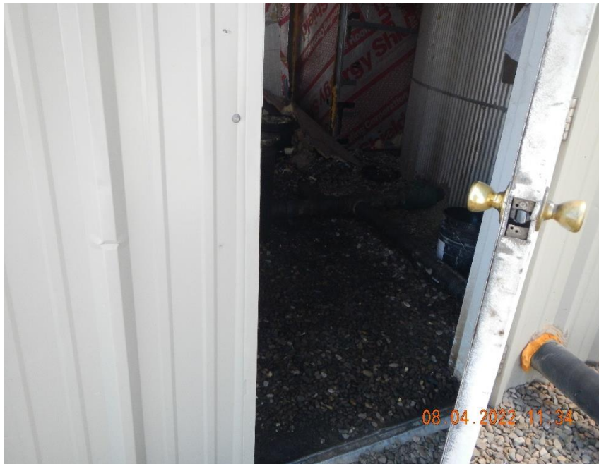
Oil stained ground and gravel inside of pump house.
