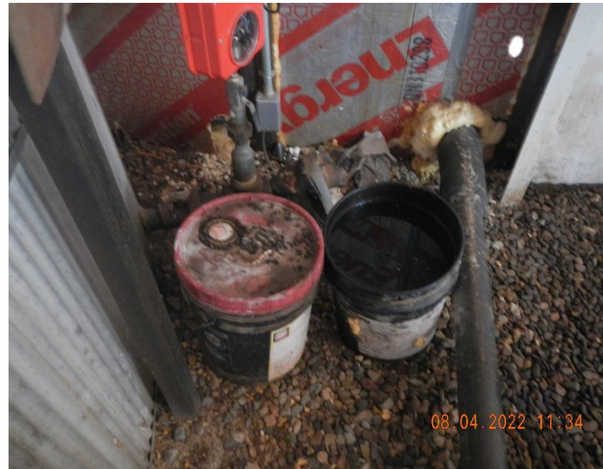
Full bucket without lid. No secondary containment.
