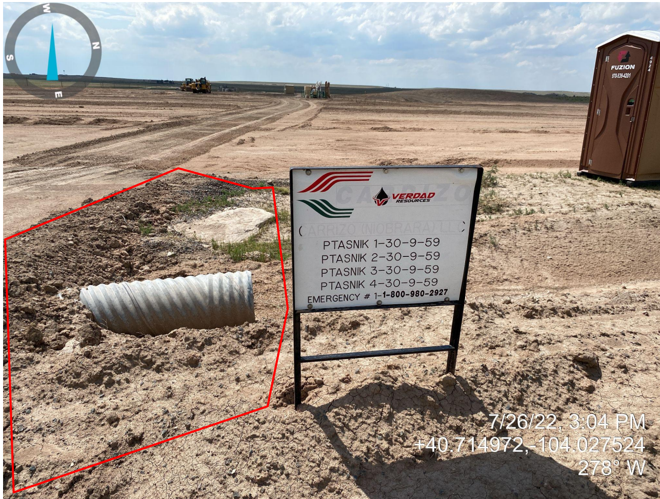
Photo 1. Location photo taken from entrance, facing west. Photo illustrates unconsolidated material around culvert (highlighted in red).
