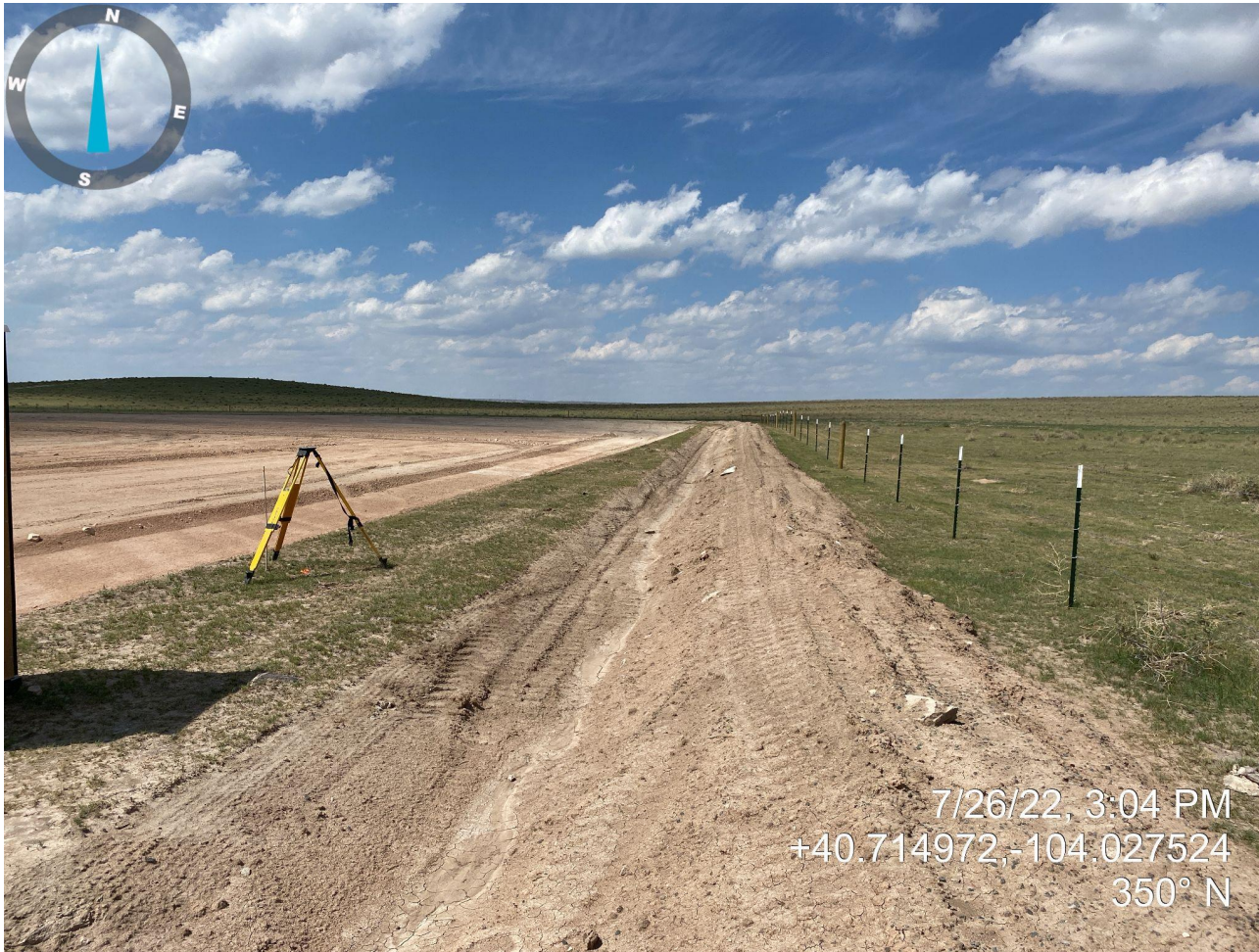
Photo 2. Location photo taken from entrance, facing north. Photo illustrates ditch and berm BMP installed during construction phase.
