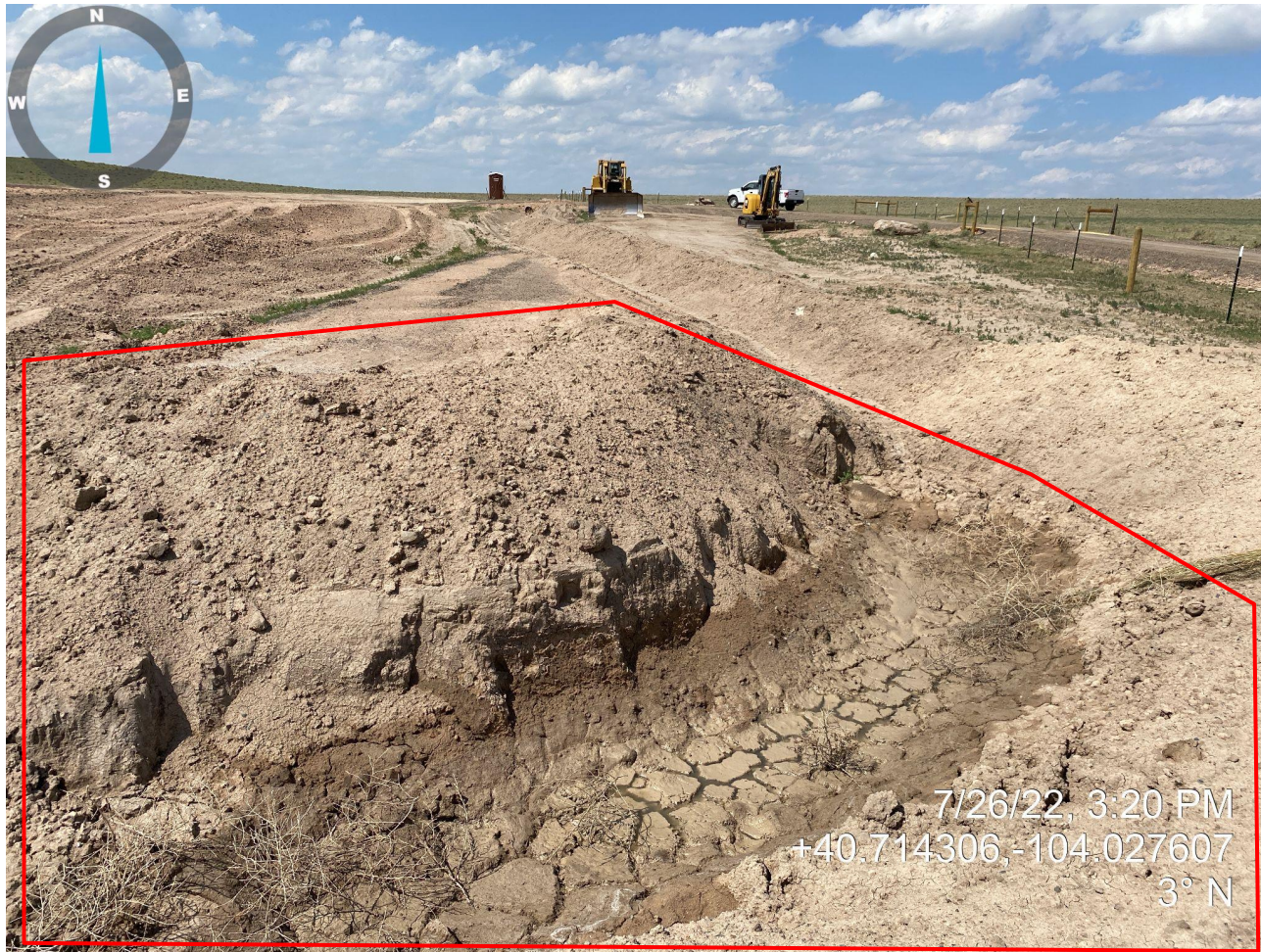
Photo 10. Ditch and berm photo taken from southeast portion of location, facing north. Photo illustrates unconsolidated material (highlighted in red).
