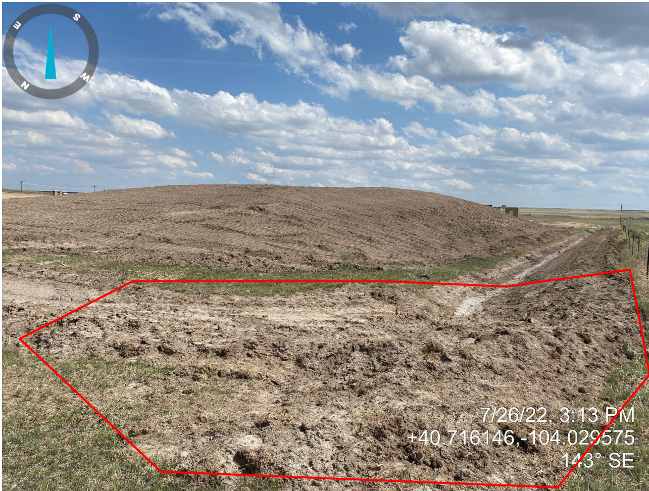
Photo 6. Location photo taken from northwestern portion, facing southeast. Photo illustrates unconsolidated material in ditch and berm BMP (highlighted in red).
