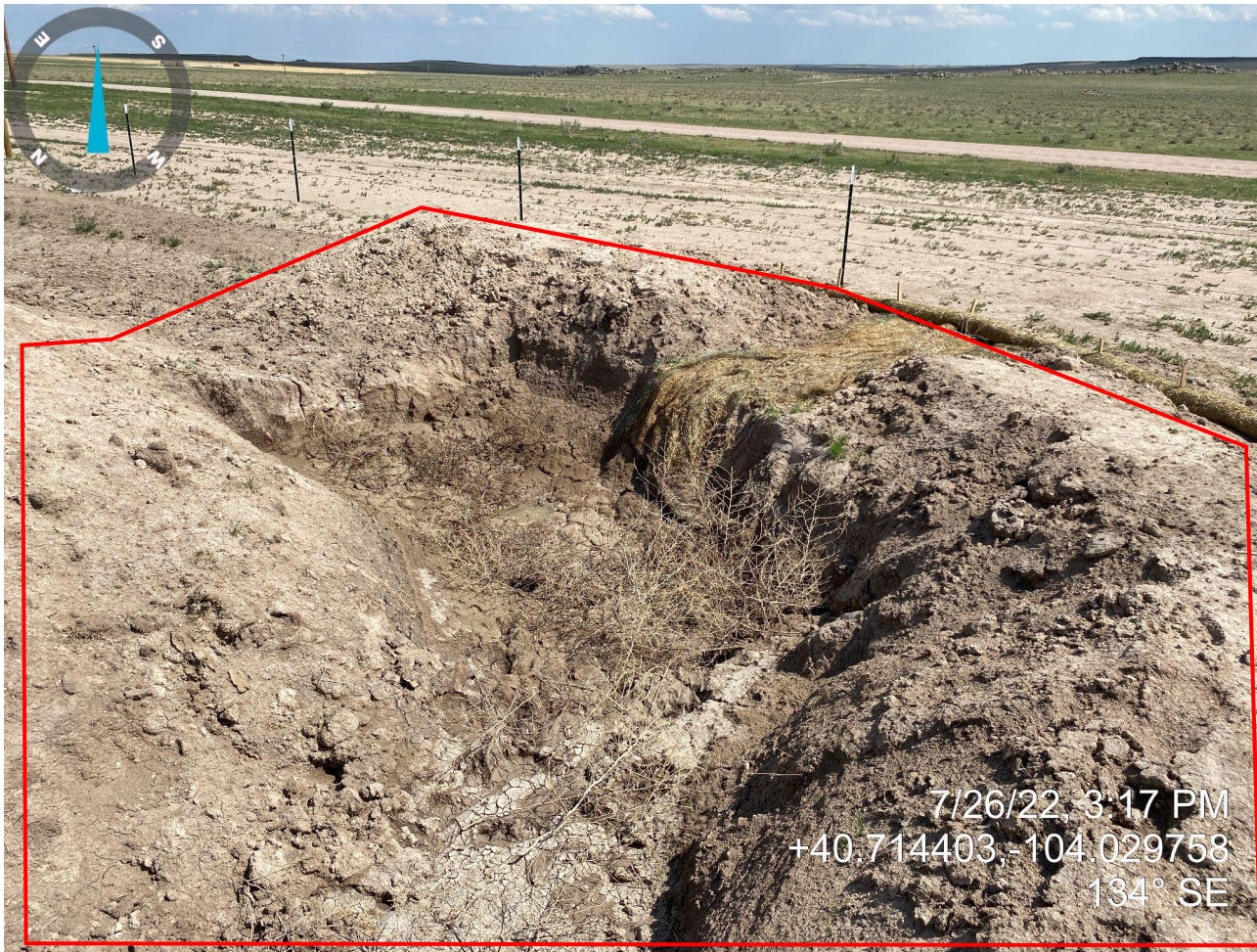
Photo 8. Sediment trap photo taken from southwest portion of location, facing southeast. Photo illustrates sediment trap walls not properly stabilized (e.g. vertical) and unconsolidated material.
