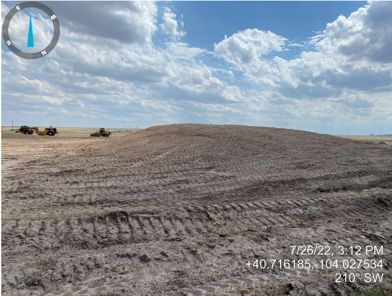
Photo 5. Location photo taken from northwestern portion, facing southwest. Photo illustrates topsoil stockpile has been temporarily stabilized with equipment tracking.
