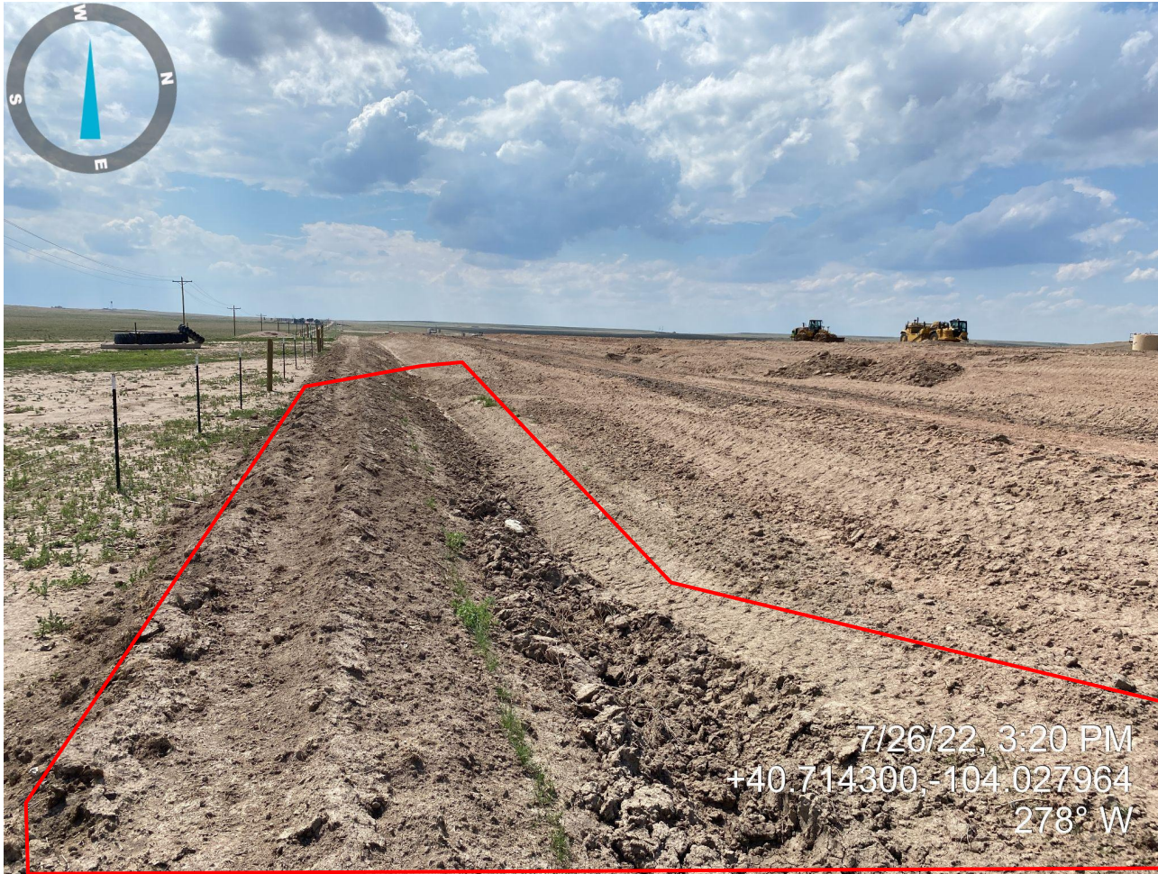
Photo 9. Ditch and berm photo taken from southern portion of location, facing west. Photo illustrates unconsolidated material in ditch (highlighted in red).
