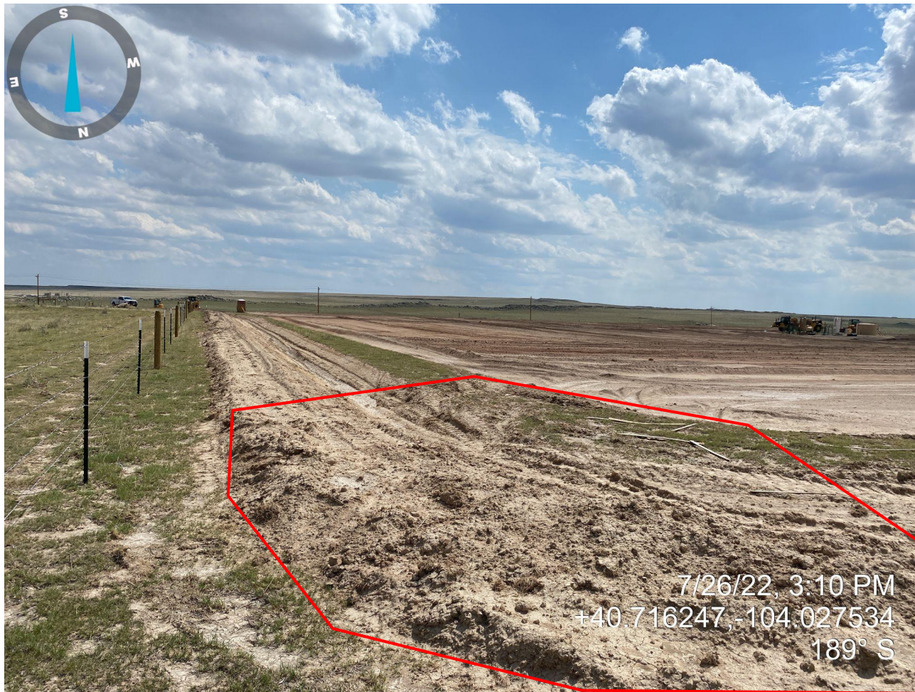
Photo 3. Location photo taken from northeastern portion, facing south. Photo illustrates unconsolidated material in ditch and berm BMP (highlighted in red).
