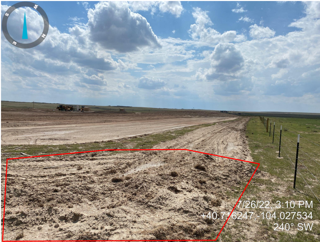
Photo 4. Location photo taken from northeastern portion, facing southwest. Photo illustrates unconsolidated material in ditch and berm BMP (highlighted in red).
