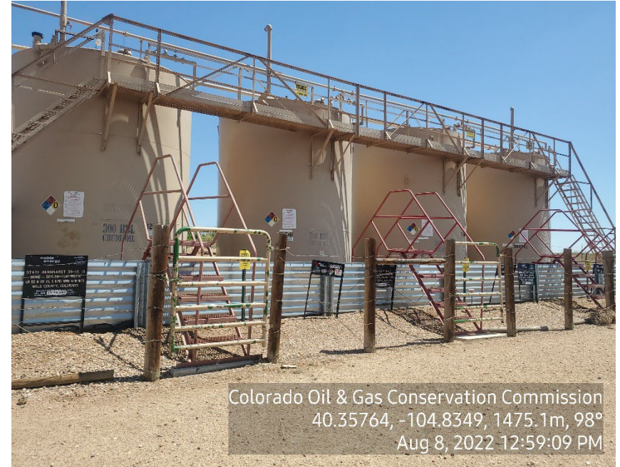
Photo 2: Centralized Tank Battery
