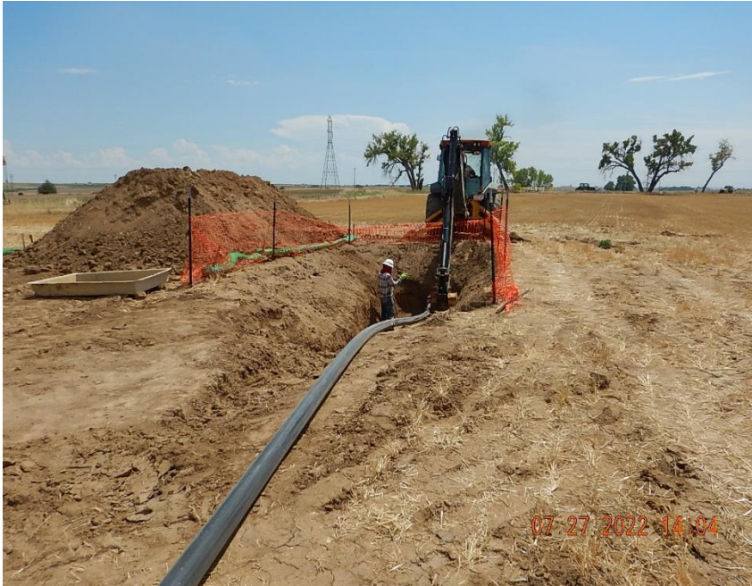
Flowline repairs being completed at North bell hole excavation. 10" OD CS pipe to 4" OD HDPE pipe transition. Approximately 800' linear feet of 4" HDPE pipe sliplined through existing 10" AJ #1 consolidation flowline (across failure point at spill ID #482628).
