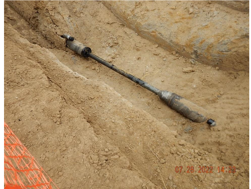
Flowline repairs being completed at south bell hole excavation. 10" OD CS pipe to 4" OD HDPE pipe transition.
