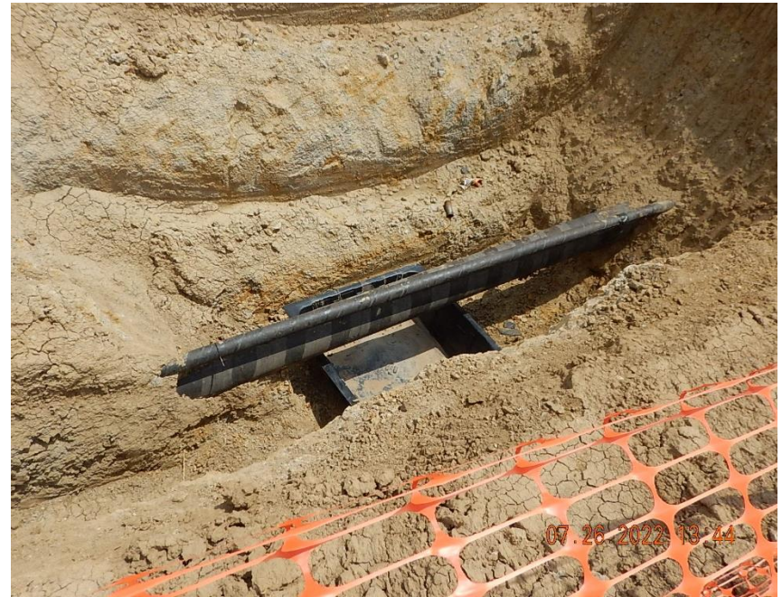
View of flowlines exposed in south bellhole excavation prior to repair; (1) 10" carbon steel AJ #1 consolidation flowline; (1) 2" carbon steel off location gas flowline.
