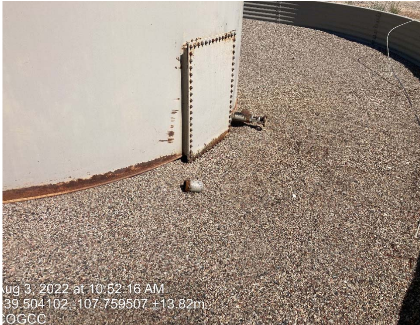
Valve missing cap/plug
