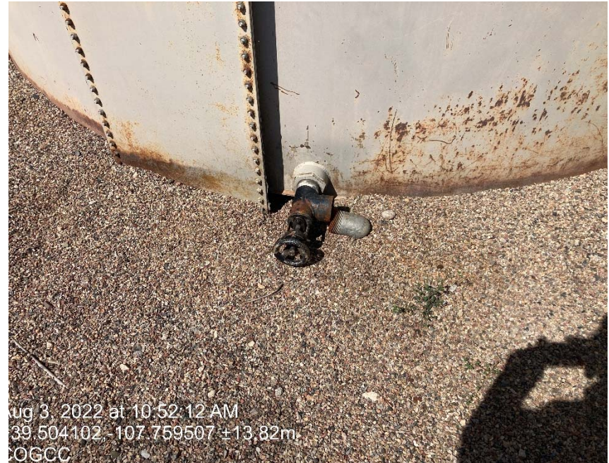
Valve missing cap/plug
