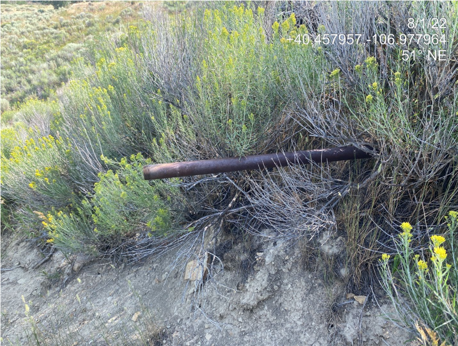
Photo 5. Photo taken from the west of the Location shows a buried pipe coming out of the fill slope of the Location.
