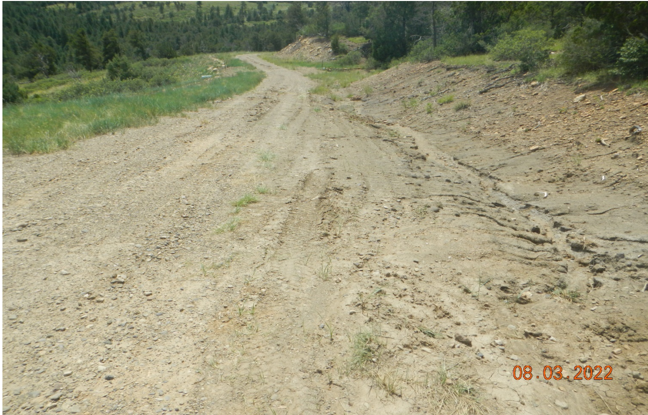
Photo 1. Facing southwest the beginning of the access road. The road has not been recontoured and reclaimed. The roadside is not stabilized and there is signs or erosion.
