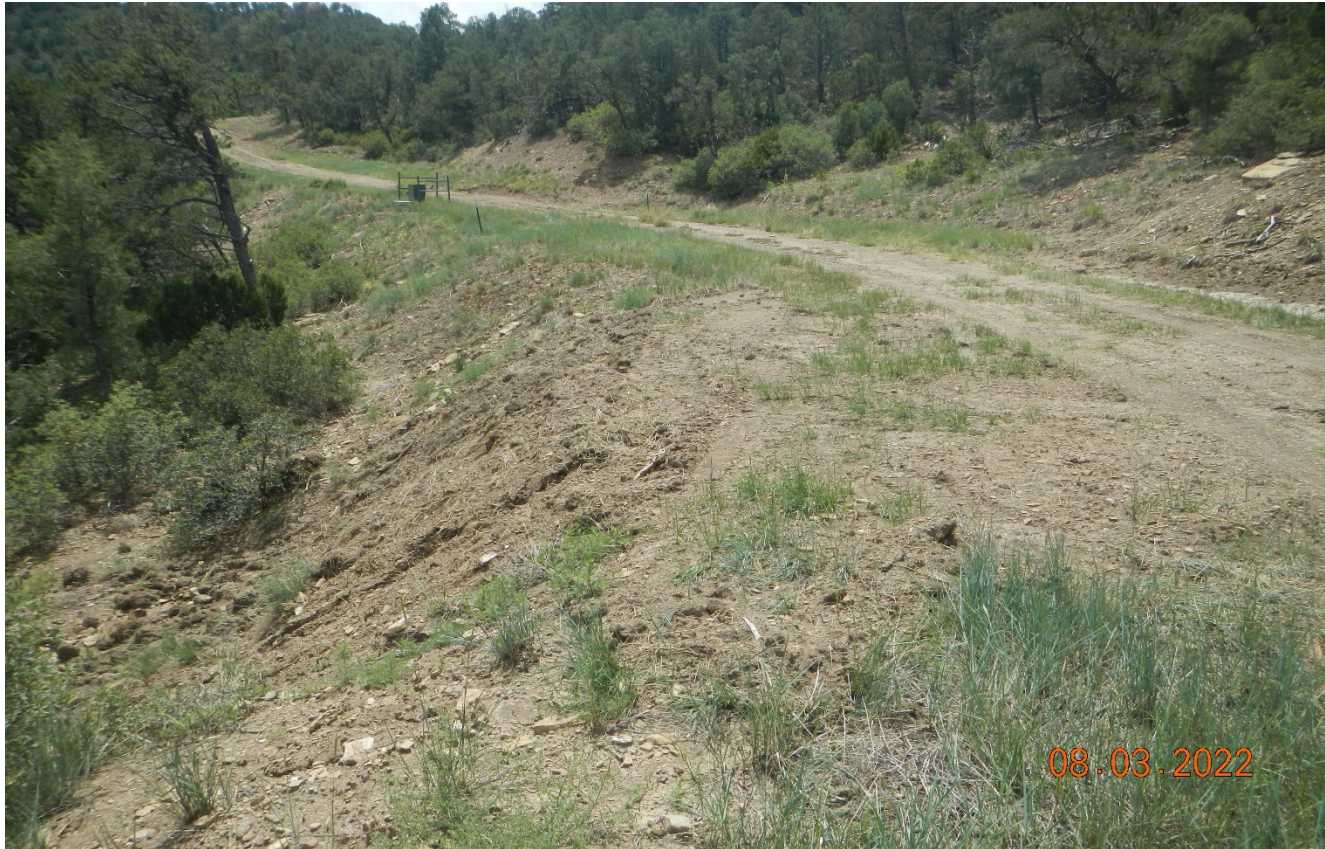
Photo 3. Facing southwest along the access road. Excavated material was placed on the fill slope of the road. Areas of disturbance need to be reclaimed.
