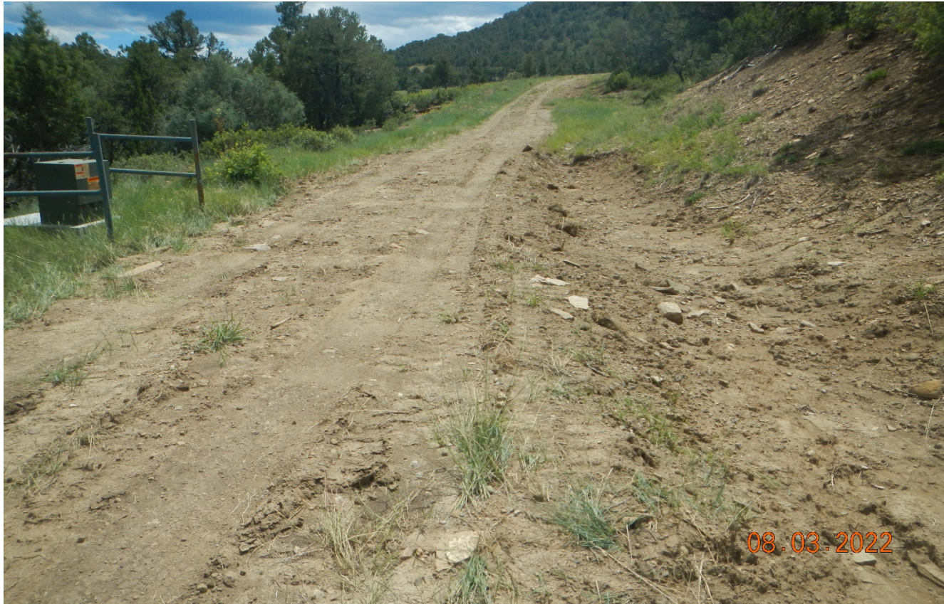
Photo 4. Facing southwest along the access road. There was recent work performed along the road. This area was partially excavated and material was placed on the road. Areas of disturbance need to be reclaimed.
