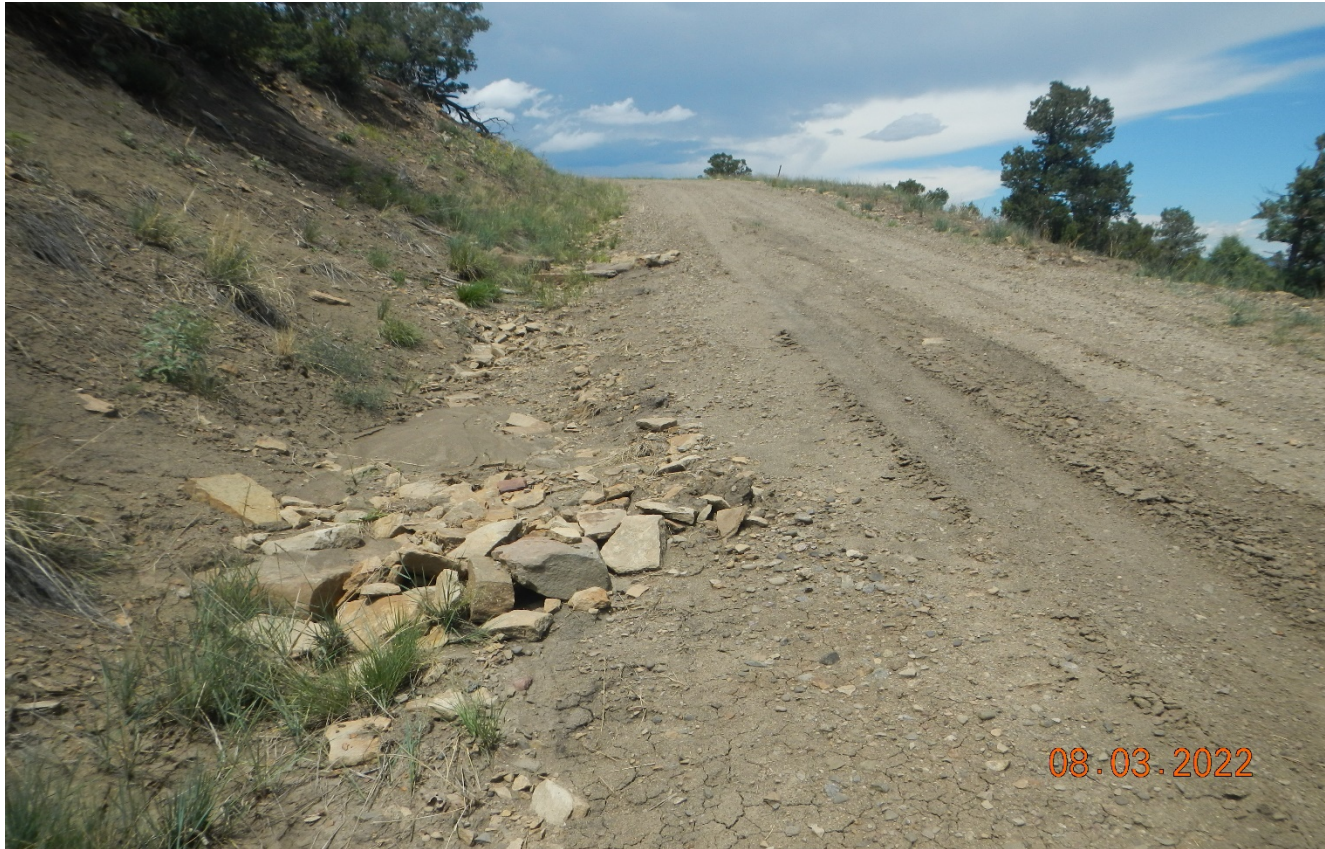
Photo 2. Facing northwest along the access road. There have been rock check dams installed however they are filled in with sediment and not properly installed.
