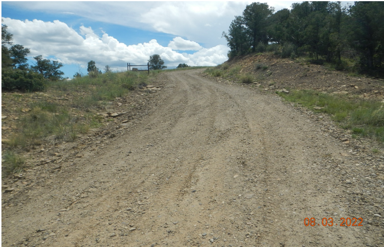
Photo 3. Facing south along the access road. The road has not been recontoured and reclaimed.
