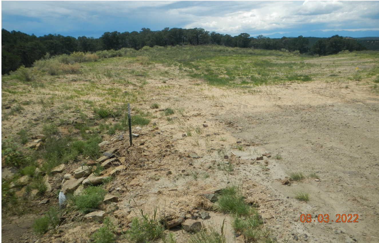
Photo 5. Facing west toward the location. The location has not been recontoured. The location was reseeded and hydromulched.
