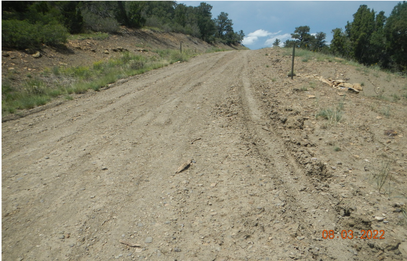
Photo 1. Facing northwest the beginning of the access road. The road has not been recontoured and reclaimed. It does not appear the road is stabilized.
