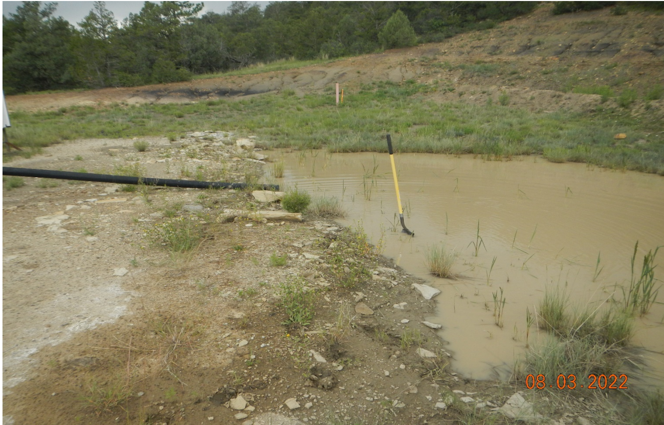
Photo 3. Facing toward the pit. The pit is shallow; less than 2 ft. deep and needs to be constructed to allow 2 ft. freeboard. Previous corrective action was not completed. Water level is above the freeboard.
