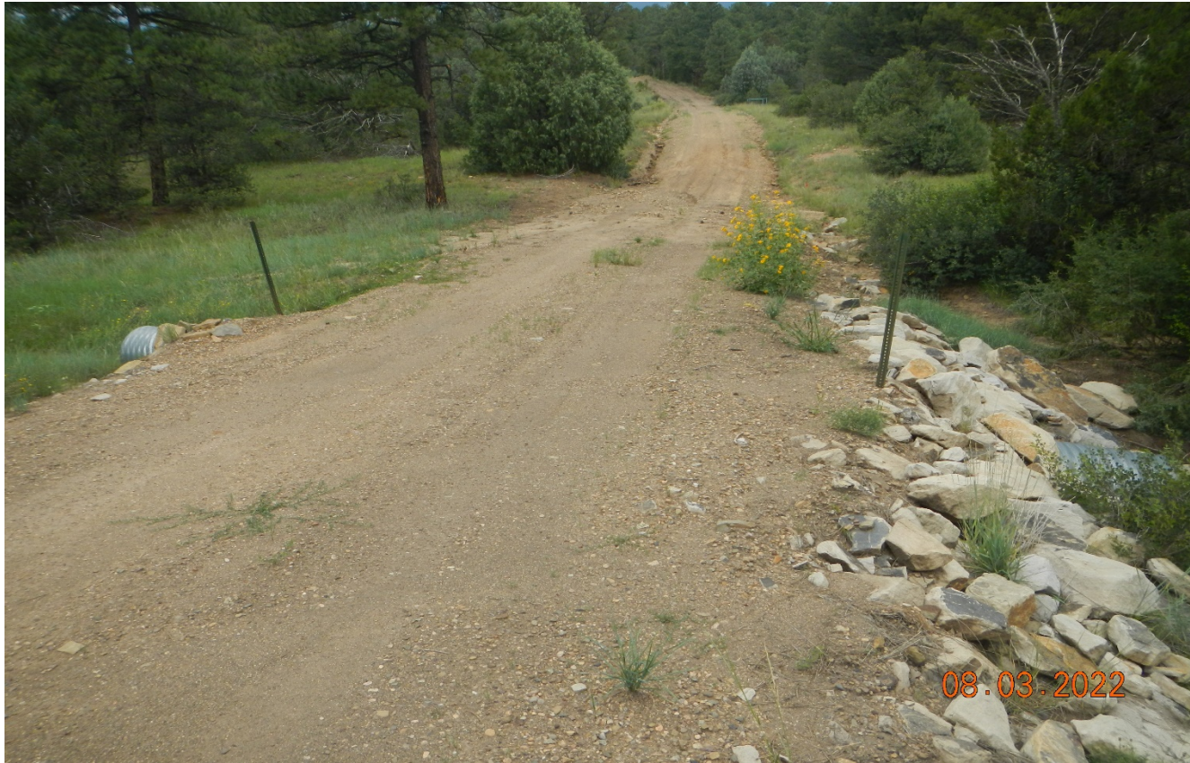
Photo 1. Facing west at the drainage crossing. This area has been repaired.
