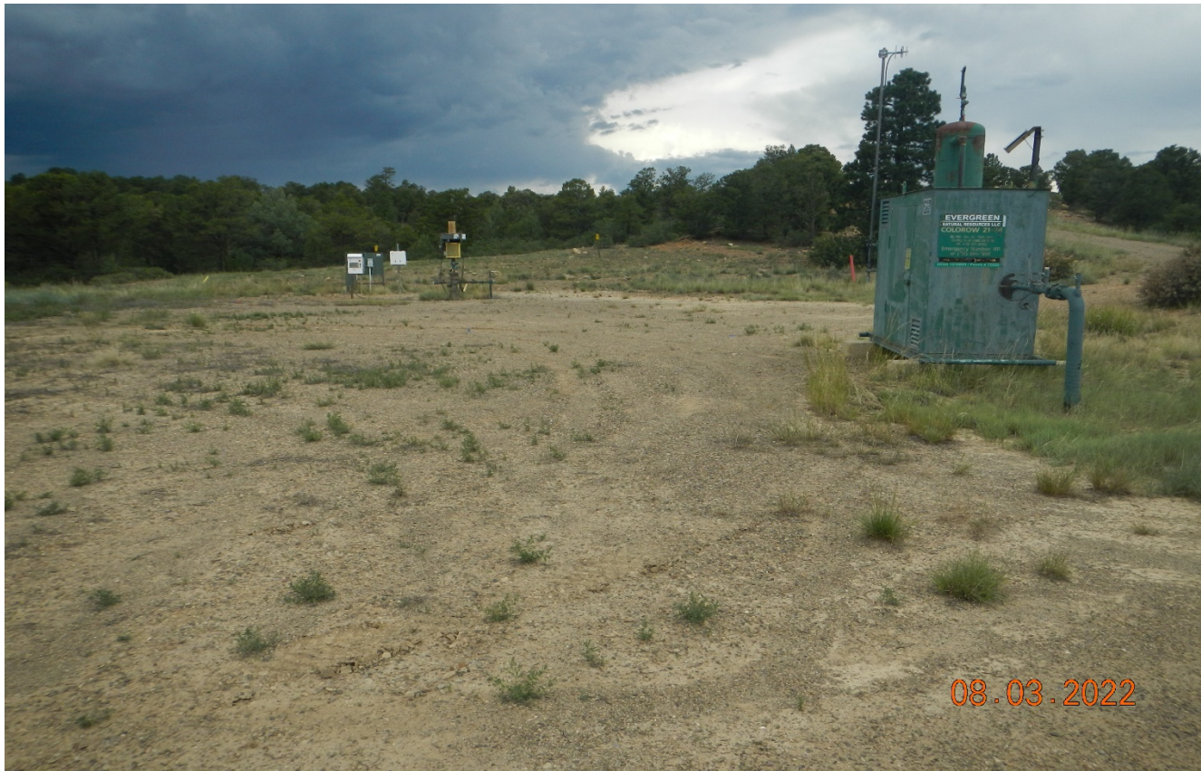
Photo 4. Facing west at the wellsite.
