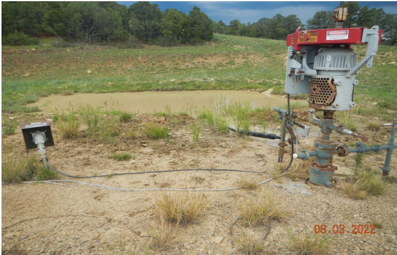
Photo 2. The water level in the pit is above 2 ft. freeboard. Did not see a freeboard marker.
