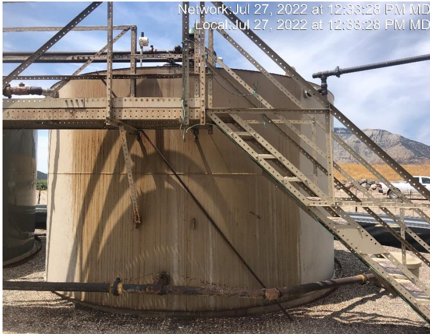
Photo #7329 Oil or condensate staining down tank.
