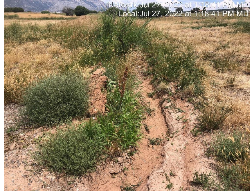
Photo #7336 No form of velocity check in ditch.
