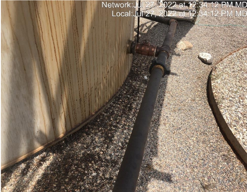
Photo #7330 Stained gravel in tank containment.
