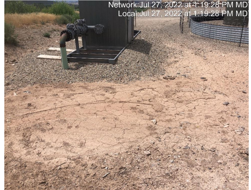
Photo #7341 Run on to location is not being controlled.
