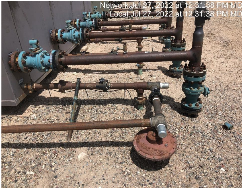
Photo #7325 2" line dumps into singular tank battery dump line.
