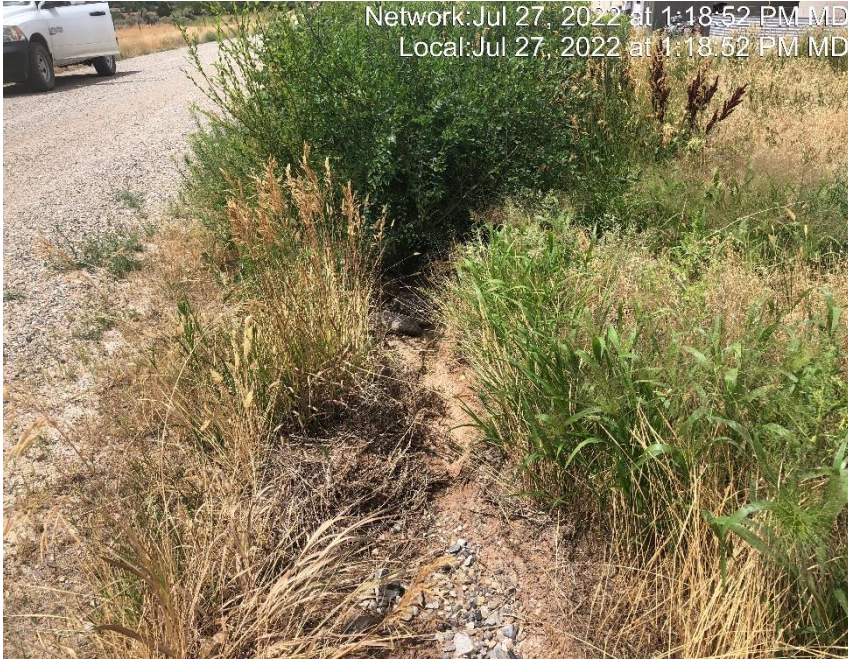
Photo #7338 No form of velocity checks in access road ditch.
