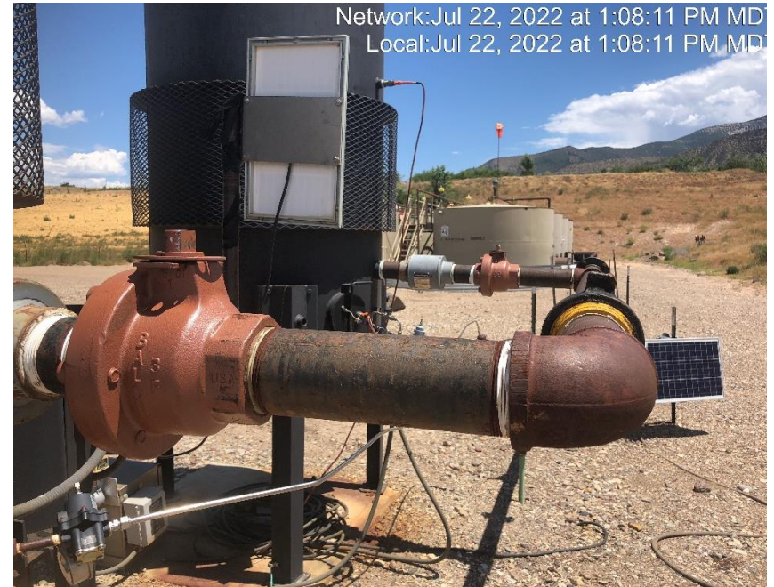
Photo #7272 combustors isolated from tank battery.
