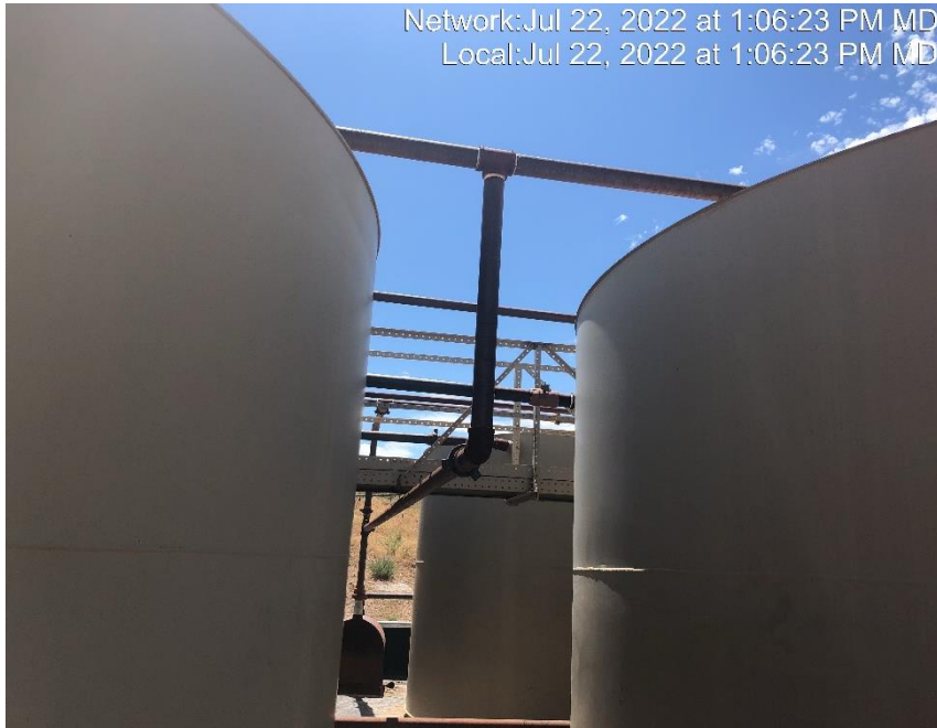
Photo #7262 Vent line from produced water tank to condensate tanks no isolation.
