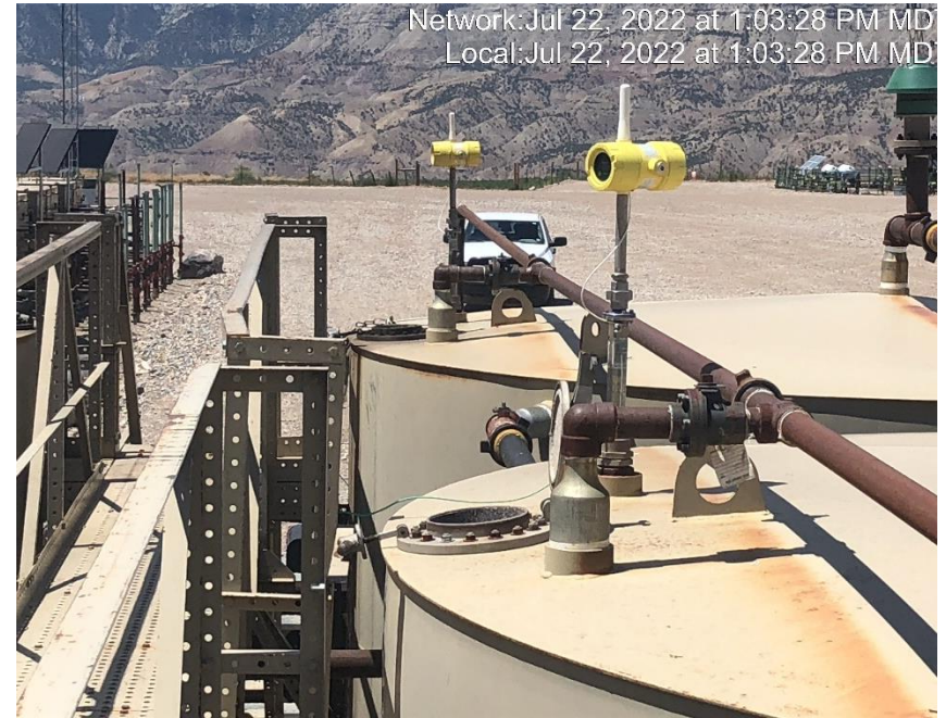
Photo #7256 Thief hatches opened for depressurizing tank battery.
