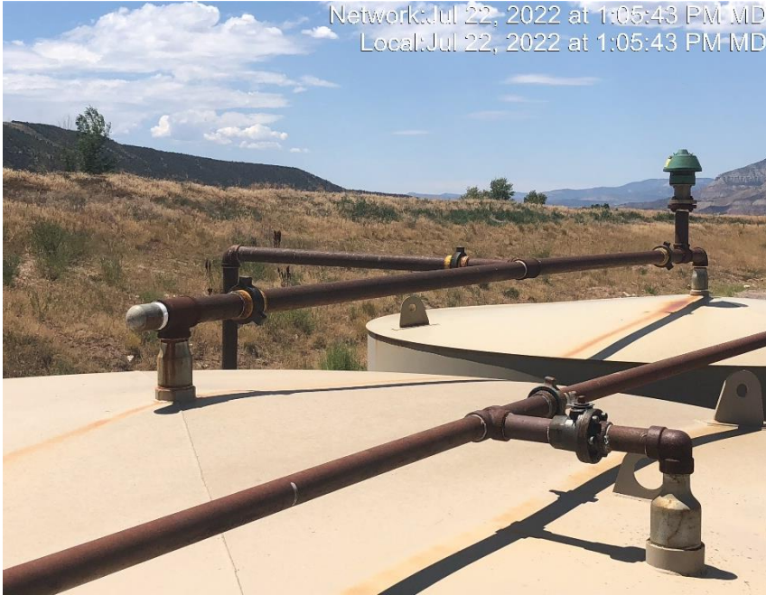
Photo #7358 Vent line on condensate side of tank battery.
