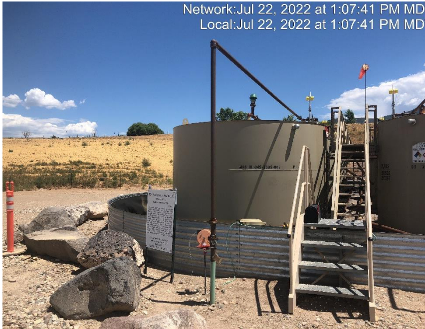
Photo #7268 Produced water tank dump line.
