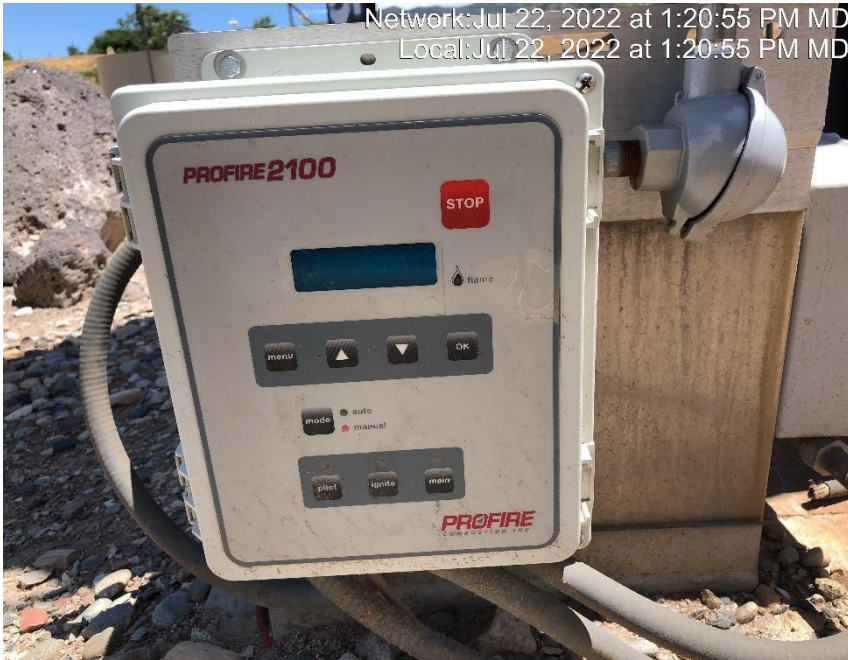
Photo #7281 Profire 2100 does not appear to be on.
