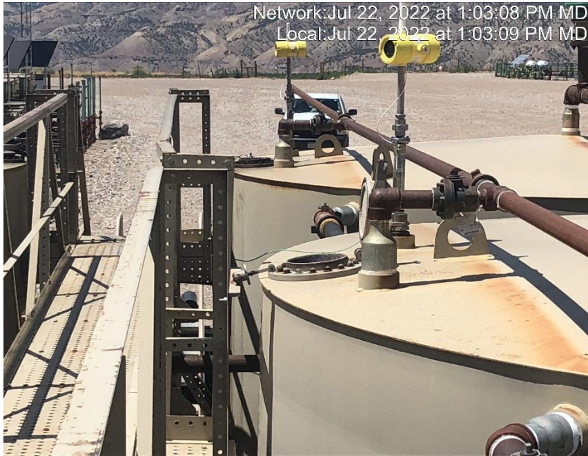
Photo #7255 Thief hatches opened for depressurizing tank battery.
