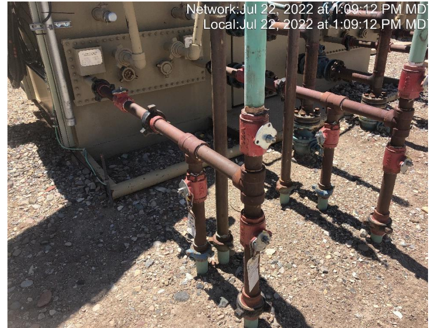
Photo #7276 23A-17-07 well blowdown line open to produced water tank and isolated from the separator.
