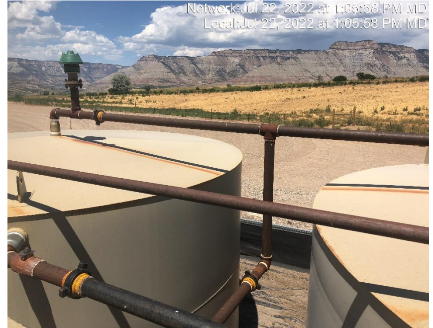
Photo #7260 Vent line on Produced water side of tank battery.
