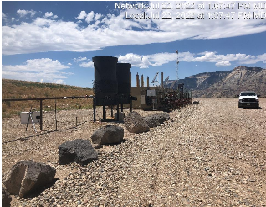
Photo #7270 Vent line coming from tank battery to combustors.
