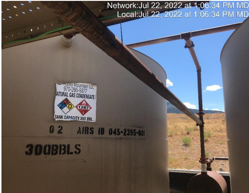
Photo #7264 Condensate tanks, AIRS ID and fluid knock out.
