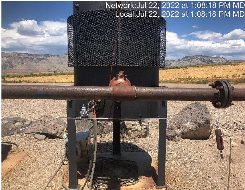
Photo #7273 Combustor isolated from tank battery.
