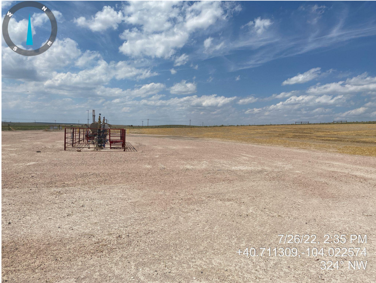
Photo 6. Location has been stabilized with road base and fenced off well head.
