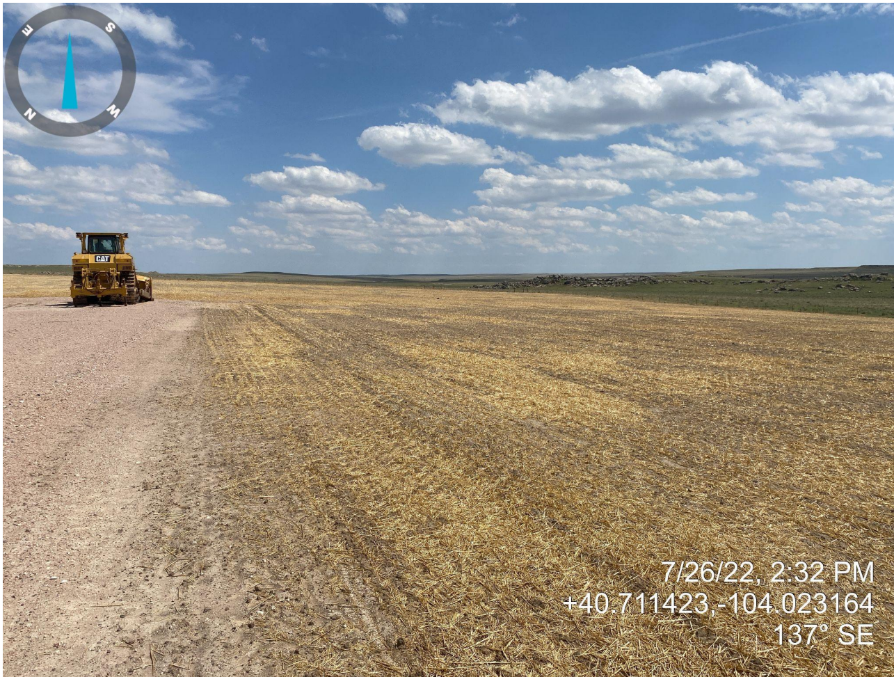
Photo 2. Photo taken from the southern portion of well pad, facing southeast. Photo illustrates interim reclamation area has been regraded with stabilized soil (straw crimped).
