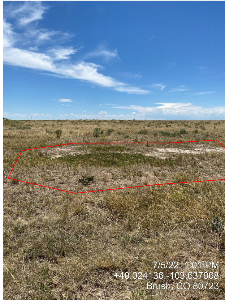
Photo 2. Location photo taken from northern portion, facing south. Subsidence (highlighted in red) observed around well location and non-uniform vegetation cover resulting in bare soil.
