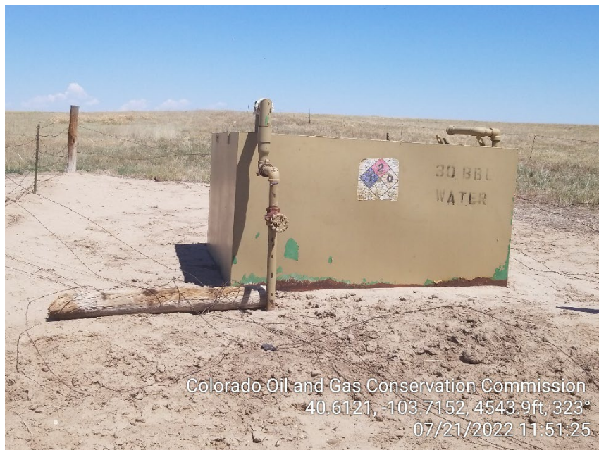
Photo 5 – Produced Water Tank
