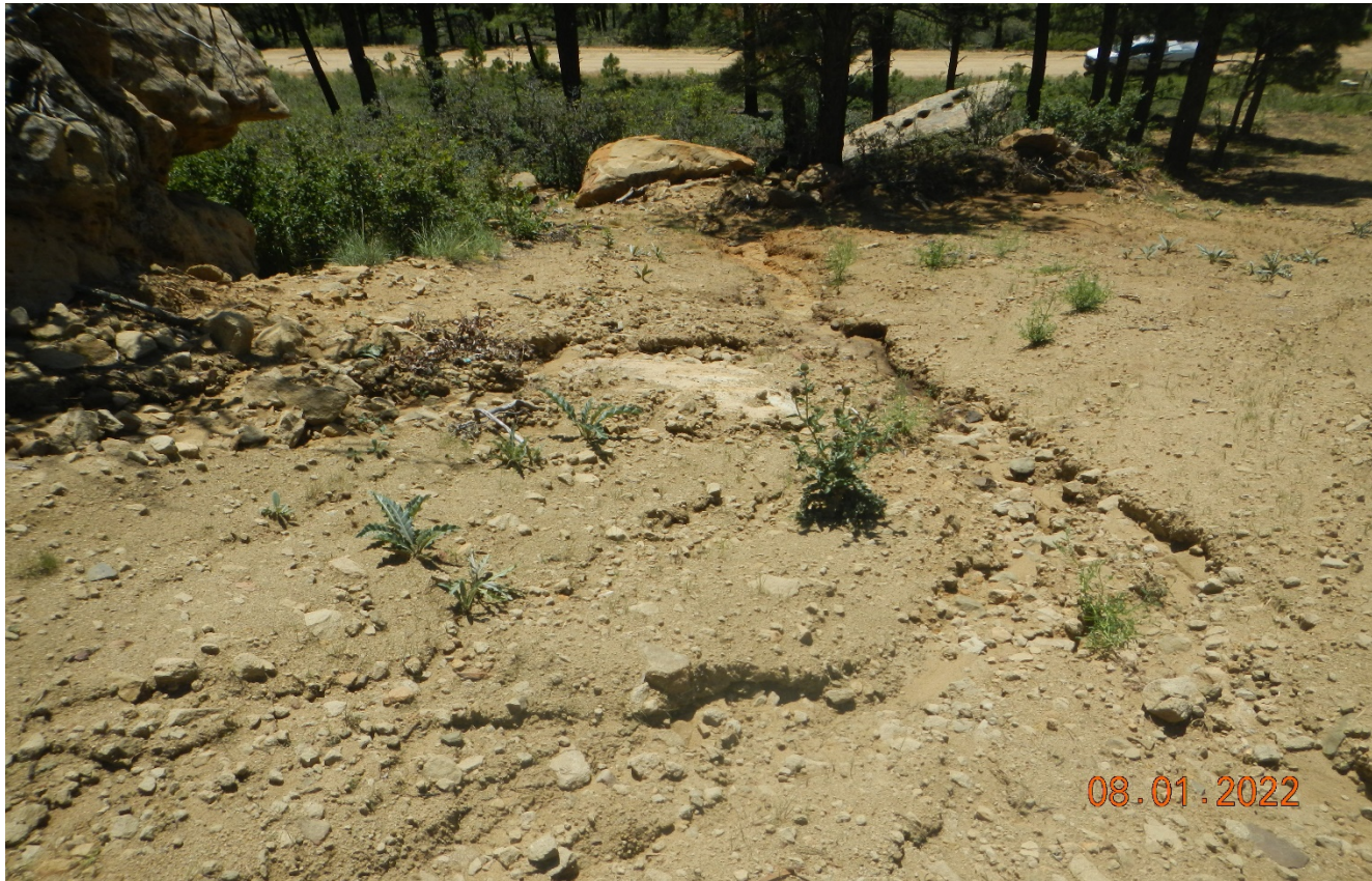
Photo 4. View of some of the erosion occurring. Additional BMP's are needed to prevent erosion.
