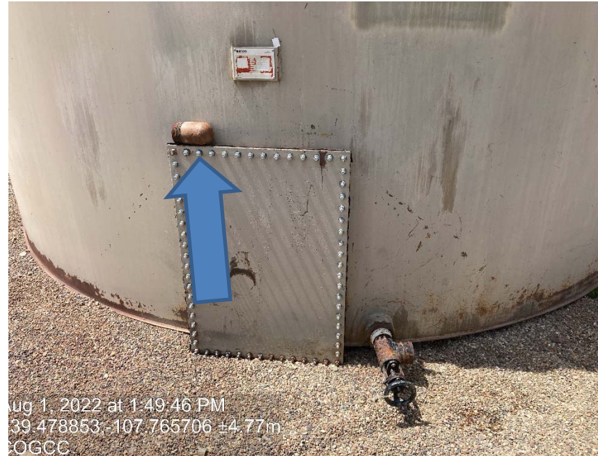
Valve on tank missing cap/plug
