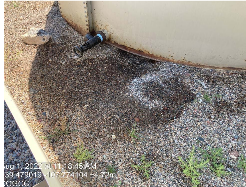
Some staining/ valve missing cap/plug
