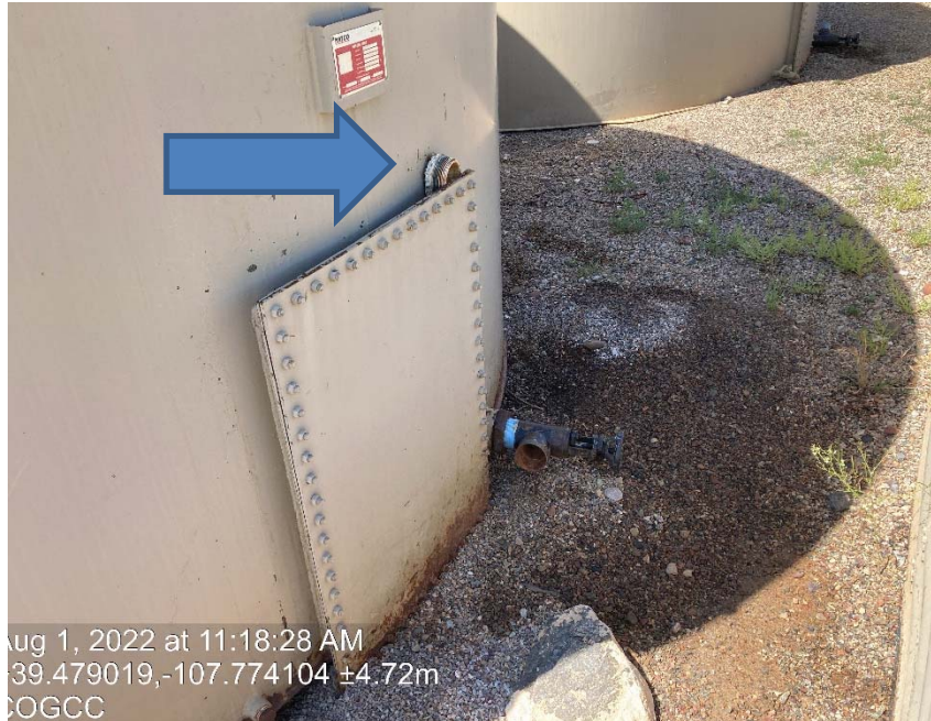
Some staining/ valve missing cap/plug
