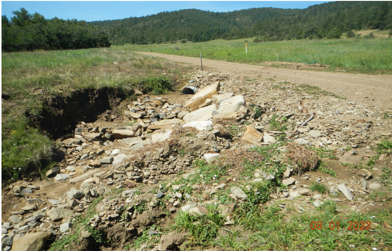
Photo 2. The culvert outlet has eroded and needs to be repaired.
