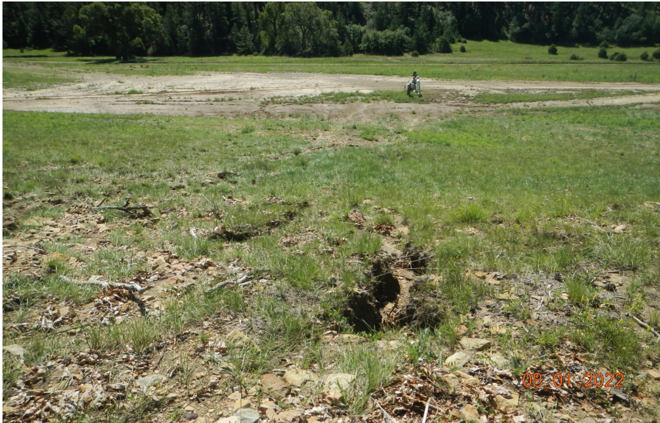
Photo 4. Facing east toward the location at the upper cut slope area. Stormwater runoff is causing erosion. This area needs to be repaired and stabilized.
