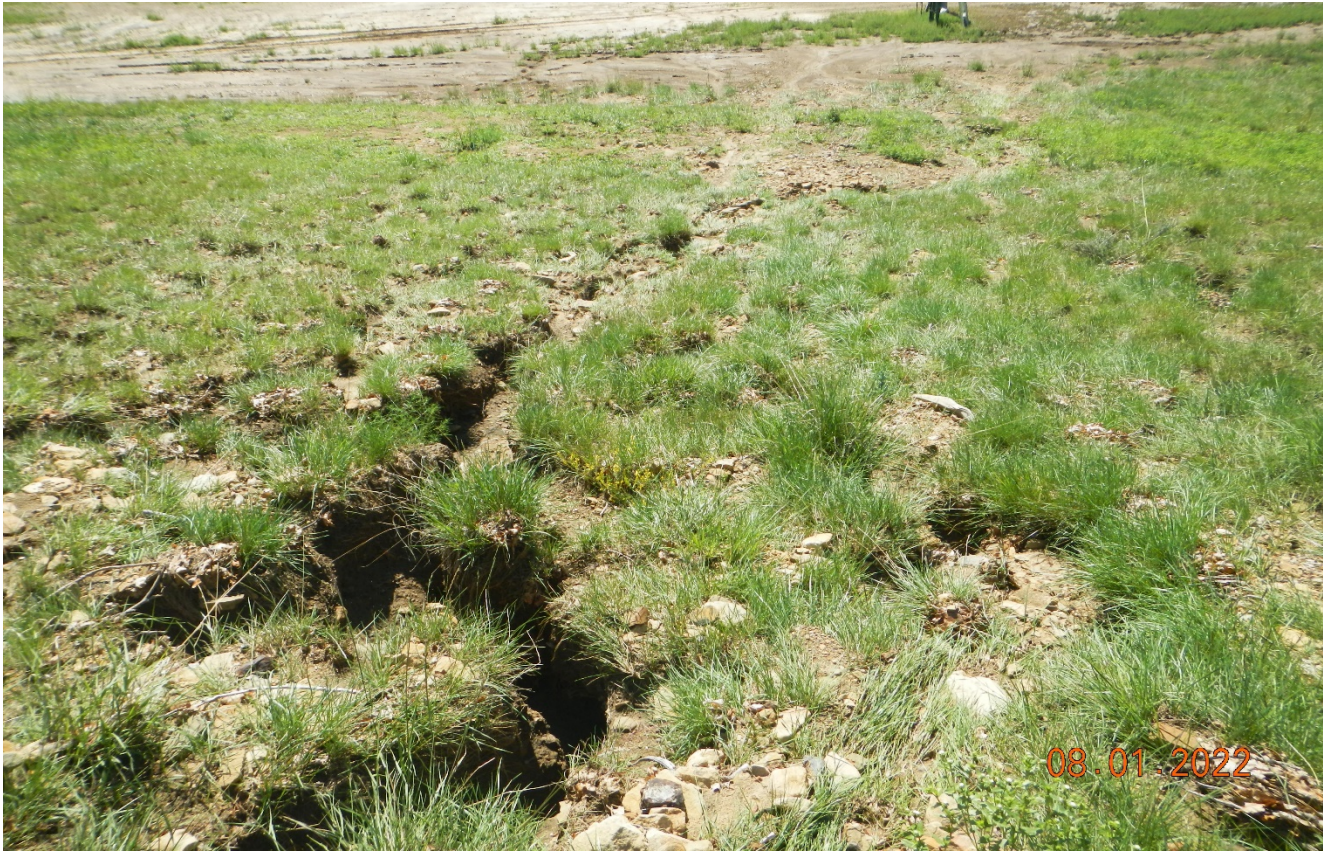
Photo 5. There is deep channeling occurring along the cut slope which must be repaired.
