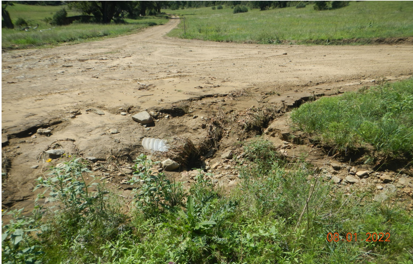
Photo 2. The culvert inlet is filled in with sediment. It appears a larger culvert is needed at this area to handle stormwater coming off the road and drainage.
