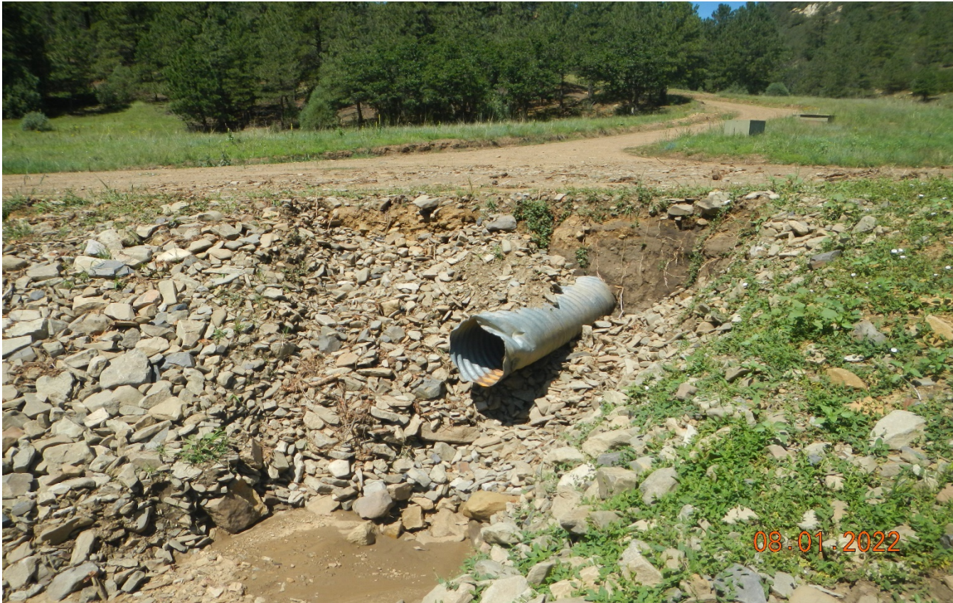
Photo 1. Facing west toward near the access road ascending the hillside. The culvert outlet has been washed out from recent storm event. It appears a larger culvert is needed along with larger rock rip/rap outlet protection.
