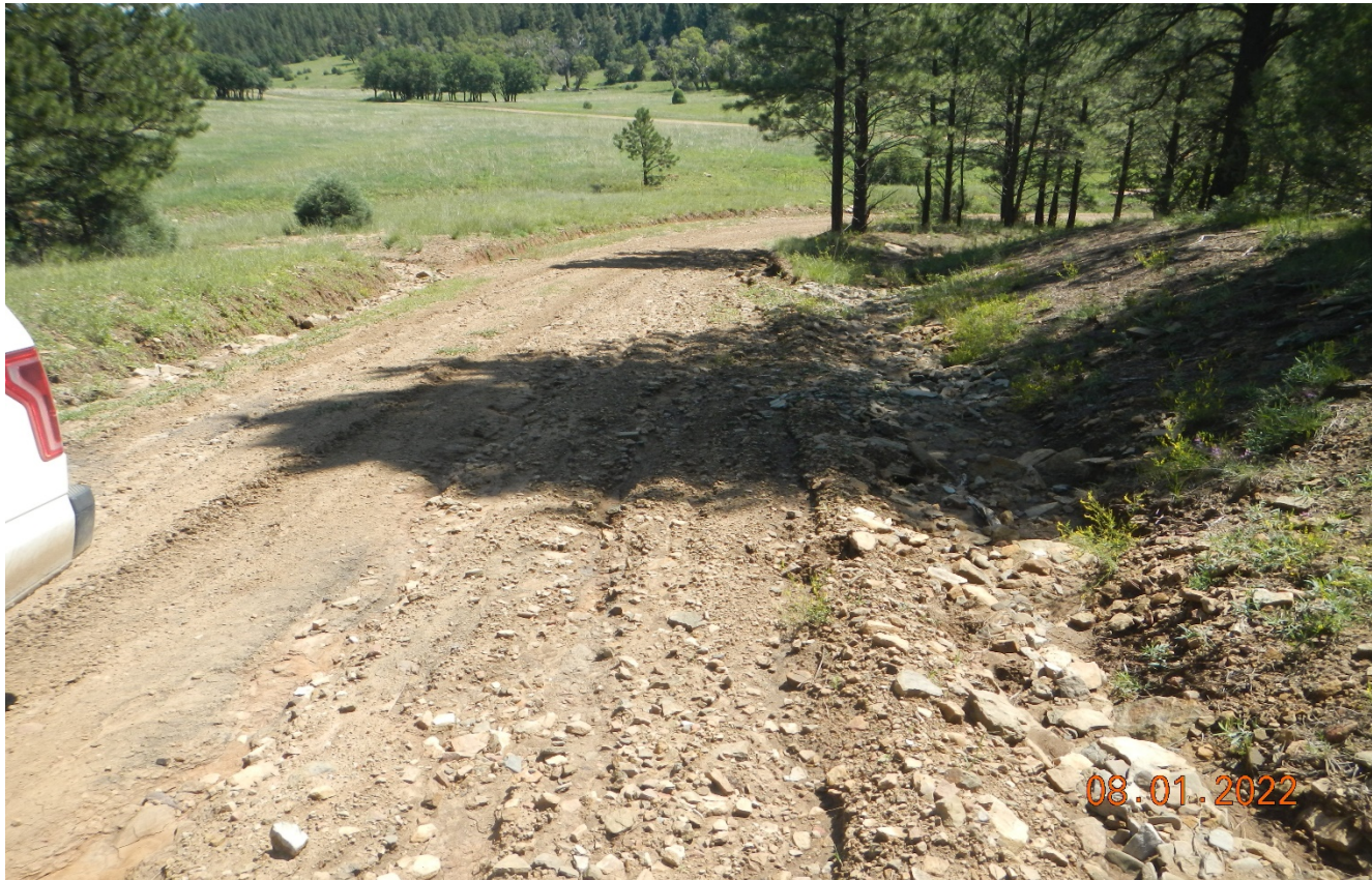
Photo 3. There are signs stormwater is flowing down the road causing erosion. This area has been a problem before. A water bar may help in this area.
