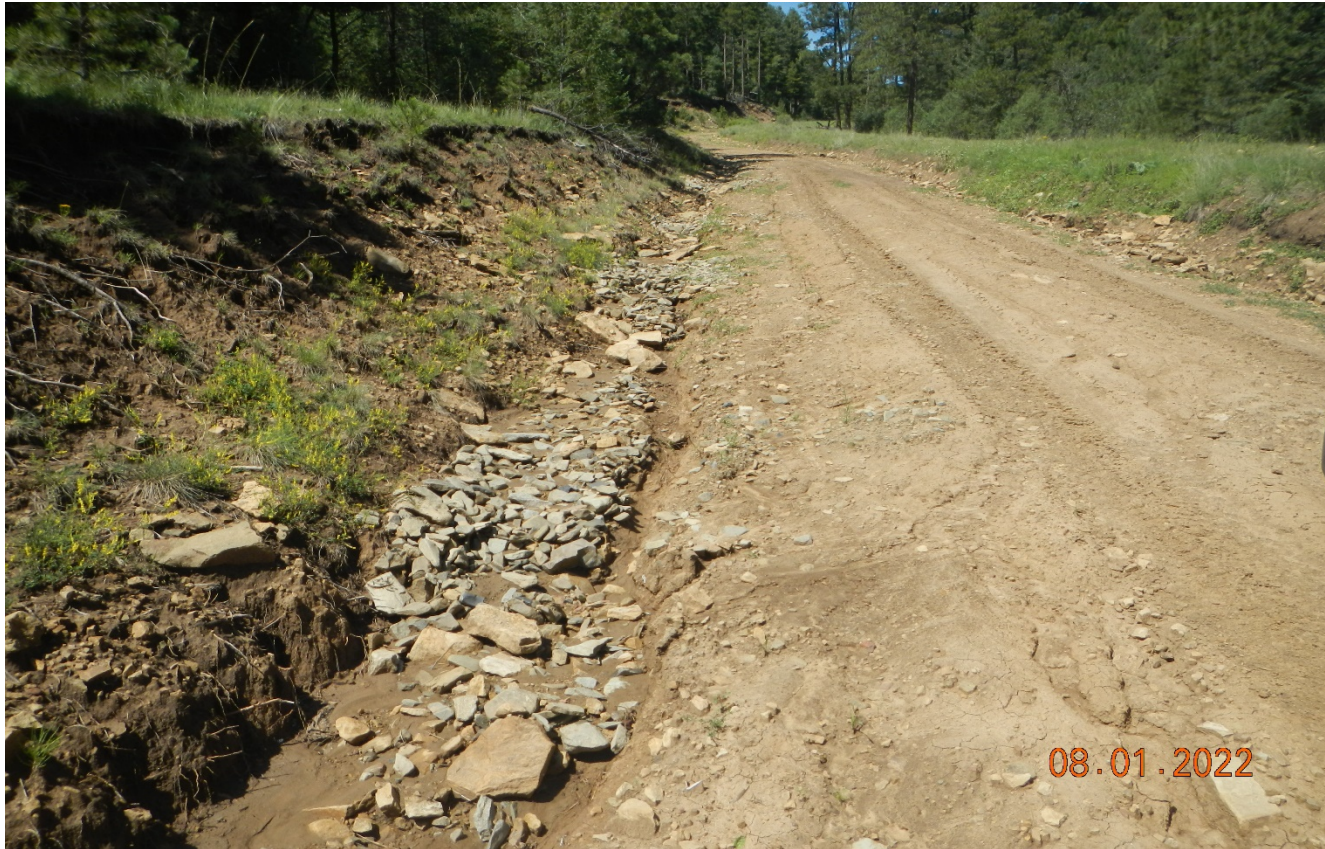
Photo 4. Facing west along the access road. Some of the rock check dams previously installed have washed out. Larger rock was likely needed.
