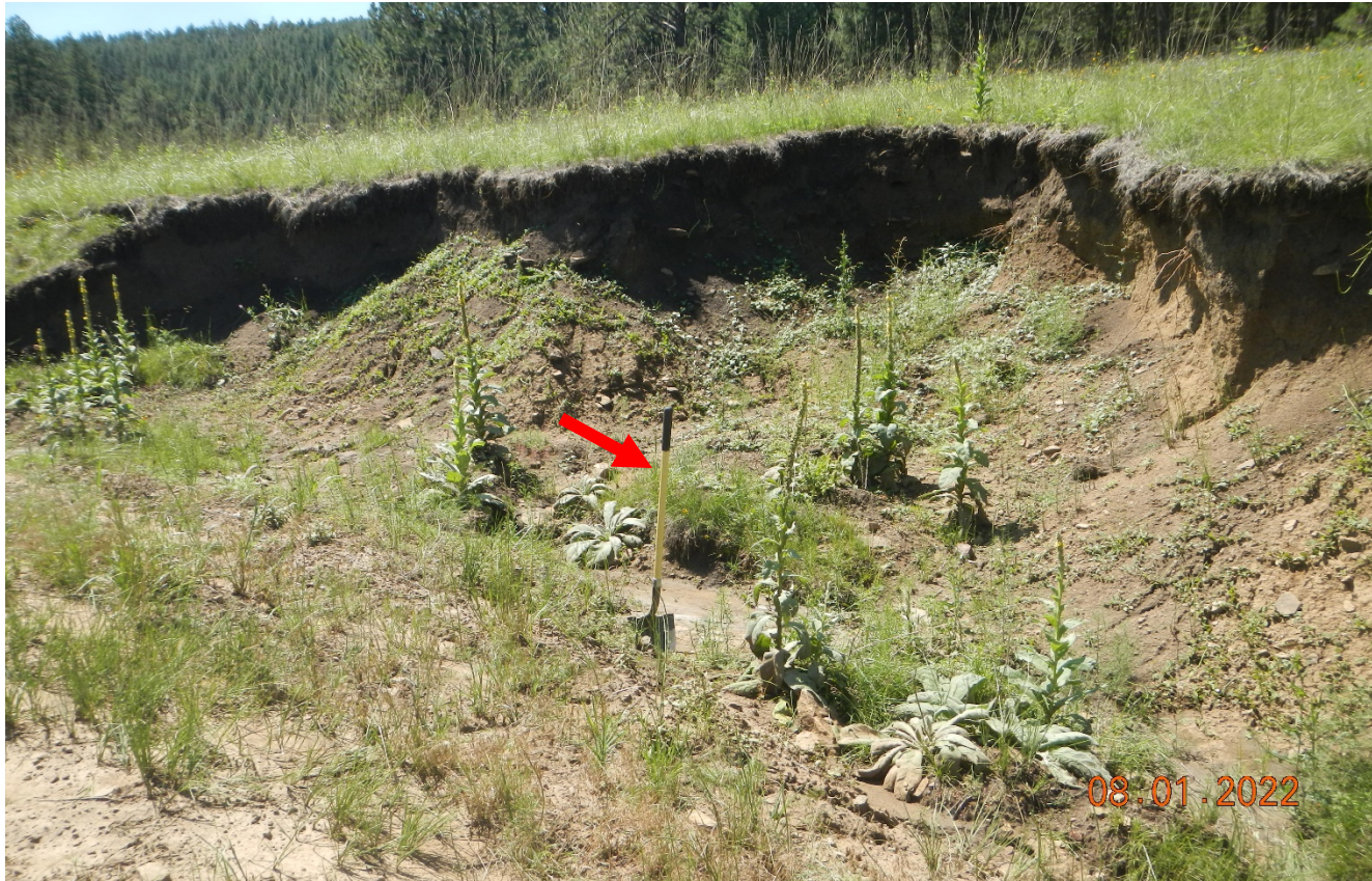
Photo 3. The side of the road is eroded and not stabilized. Erosion head cutting is continuing to occur further back. This area needs to be repaired and stabilized. Previous corrective action not completed. Red arrow points to 4.5 ft. shovel. Lat/Long:36.99952,-104.83425. There are also noxious shown in the photo.
