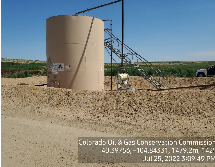
Photo 3: Tank Battery
