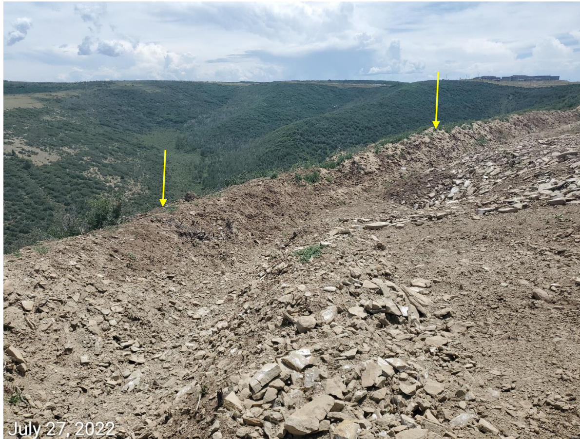
Photo 2: Photos examples showing topsoil remains in use as part of the Locations perimeter stormwater controls, specifically.
