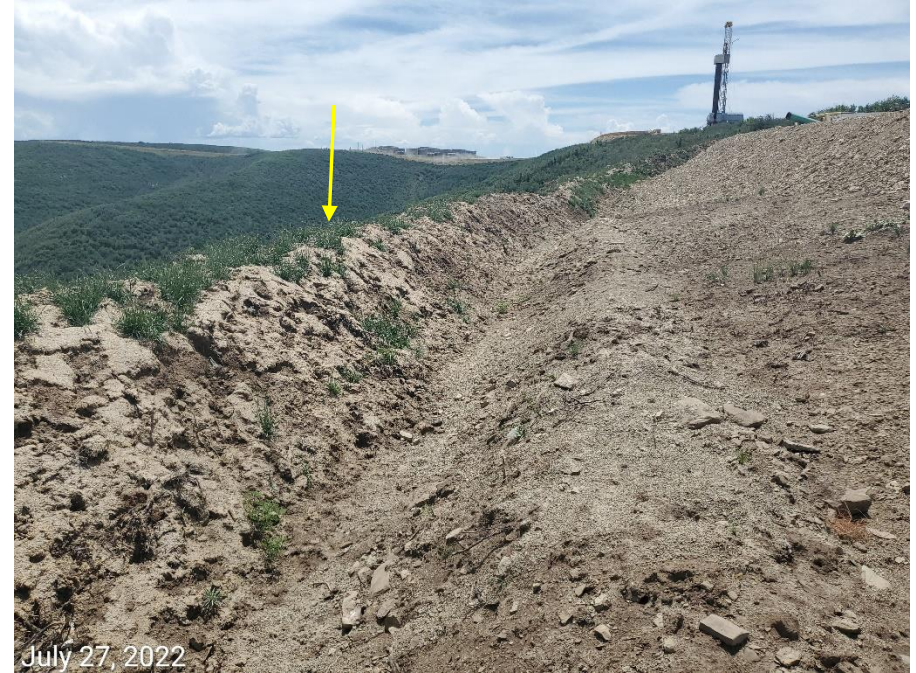
Photo 1: Photo taken from the perimeter stormwater ditch. Photo example showing topsoil (yellow arrow) in use as part of stormwater controls (ditch/berm) to manage runoff on the Location.
