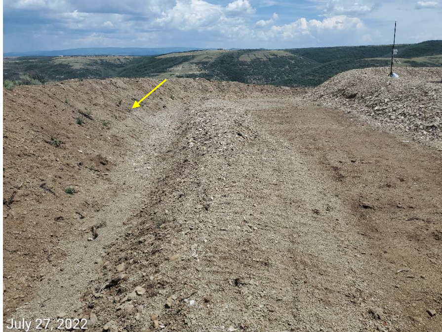
Photo 1: Photo taken from the perimeter stormwater ditch. Photo example showing topsoil (yellow arrow) in use as part of stormwater controls (ditch/berm) to manage runoff on the Location.
