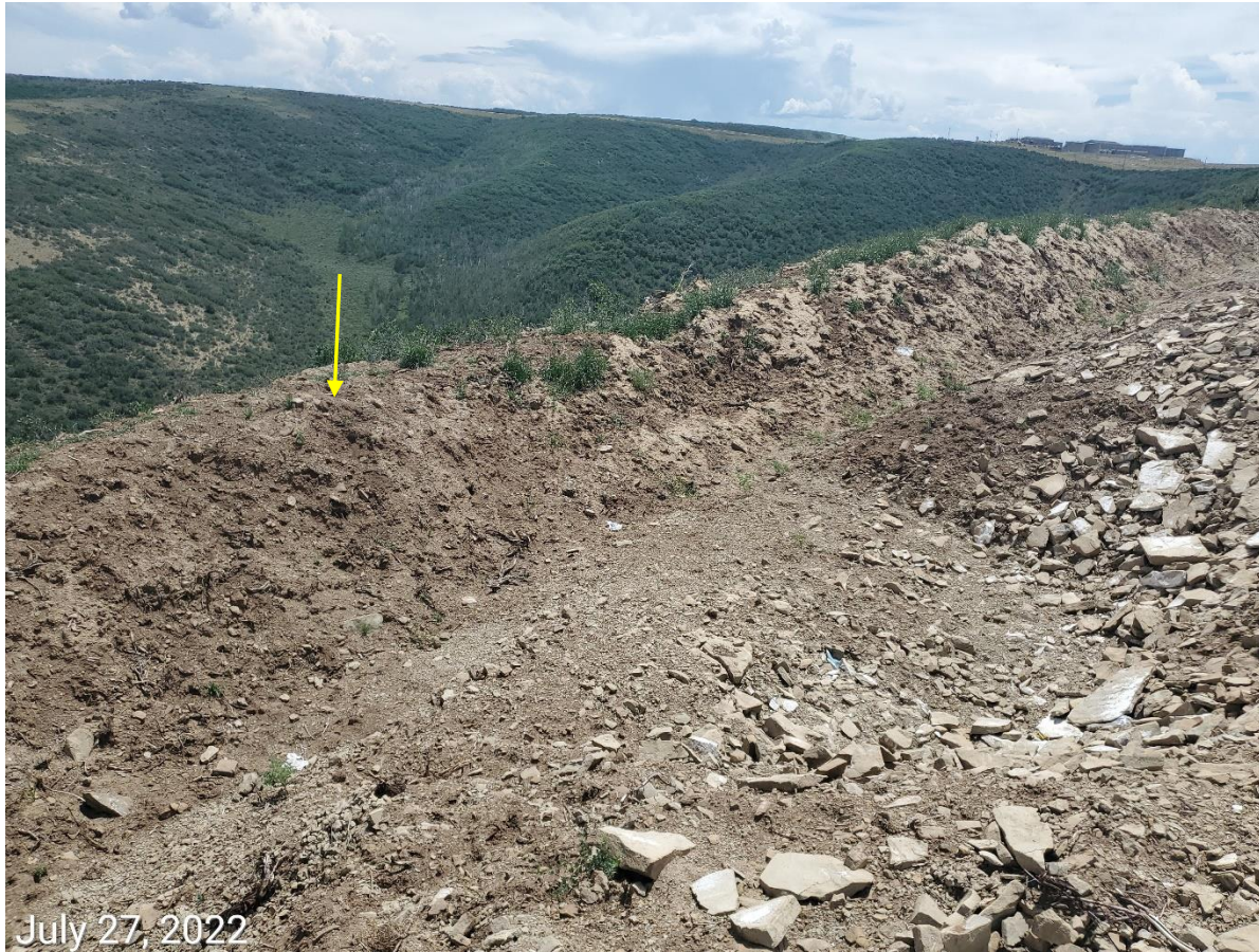
Photo 3: Photos examples showing topsoil remains in use as part of the Locations perimeter stormwater controls, specifically, the sediment trap on the east end of the Location. Photo also shows control has not been constructed with an engineered outlet to allow for proper stormwater discharge.
