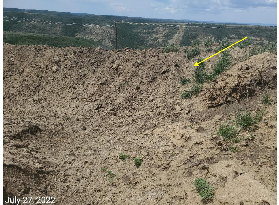
Photo 5: Photos examples showing topsoil remains in use as part of the Locations perimeter stormwater controls, specifically, one of the three sediment traps on the Location. Photo also shows control has not been constructed with an engineered outlet to allow for proper stormwater discharge.
