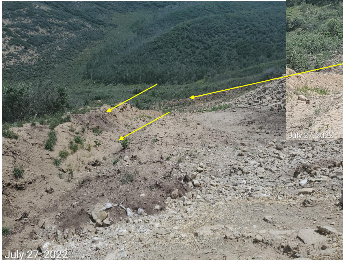
Photo 6: Additional photo example showing topsoil in use as part of the perimeter's ditch and berm, as well as the sediment traps. See comments under photo 6.
