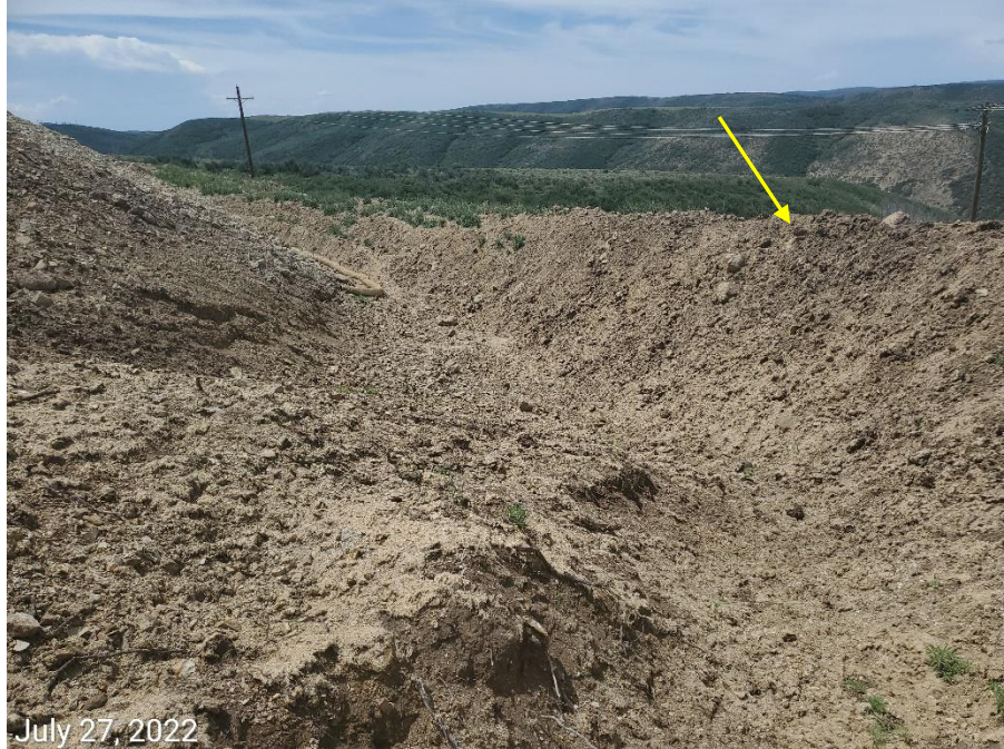
Photo 5: Photos examples showing topsoil remains in use as part of the Locations perimeter stormwater controls, specifically, one of the three sediment traps on the Location. Photo also shows control has not been constructed with an engineered outlet to allow for proper stormwater discharge.
