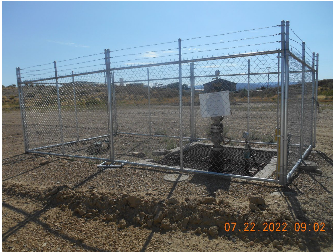
Injection wellhead. Temporarily abandoned
