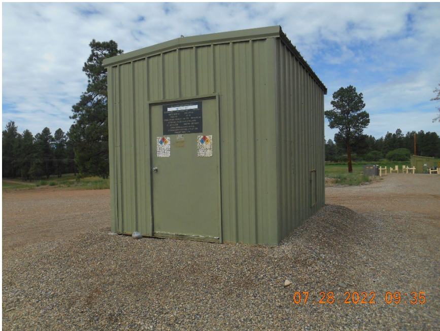
Injection wellhead inside housing
