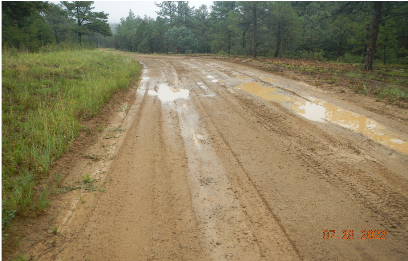
Photo 2. Facing south along the access road. There are areas where stormwater is pooling on the road causing widening of the road. This area needs additional stabilization. Approximate Lat/Long:37.24515,-104.68856
