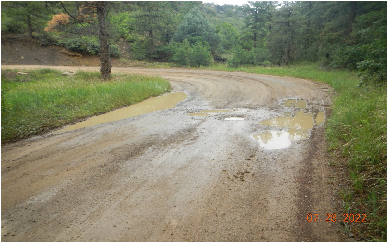
Photo 1. Facing south along the access road. There are areas where stormwater is pooling on the road causing widening of the road. This area needs additional stabilization. Approximate Lat/Long:37.23652,-104.69804
