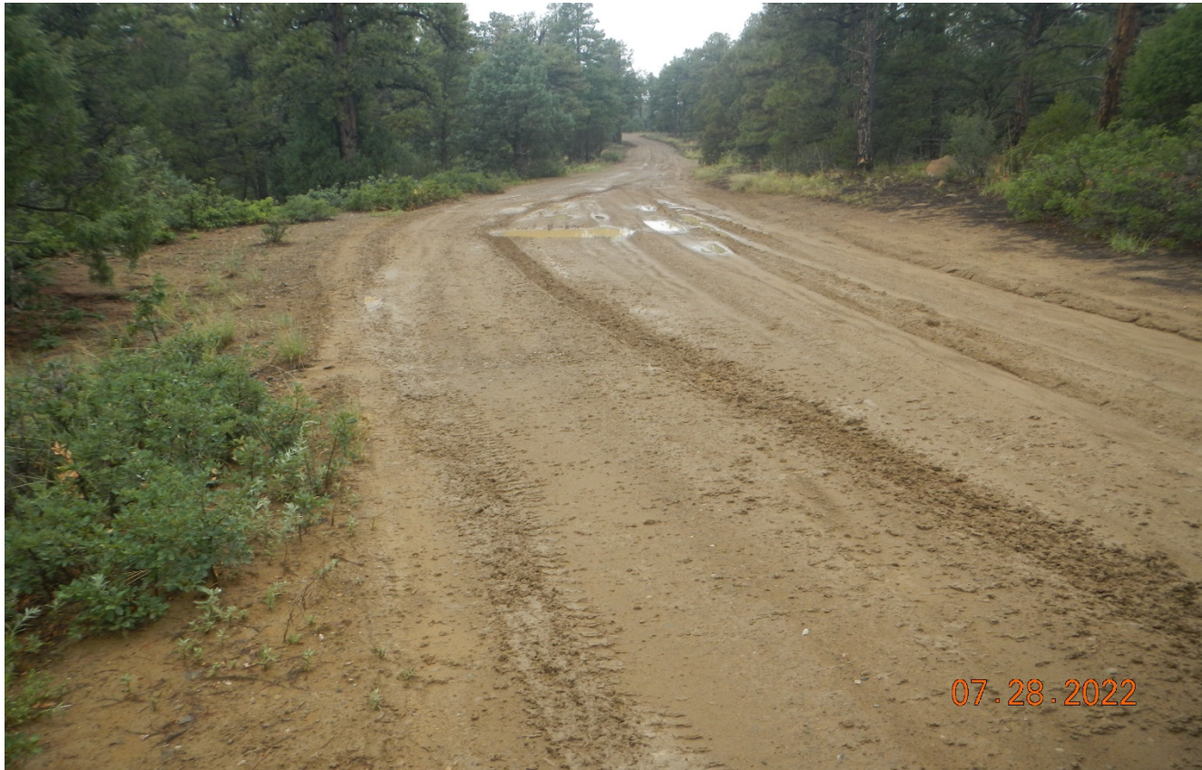
Photo 2. Facing south along the access road. There are areas where stormwater is pooling on the road causing widening of the road. This area needs additional stabilization.
