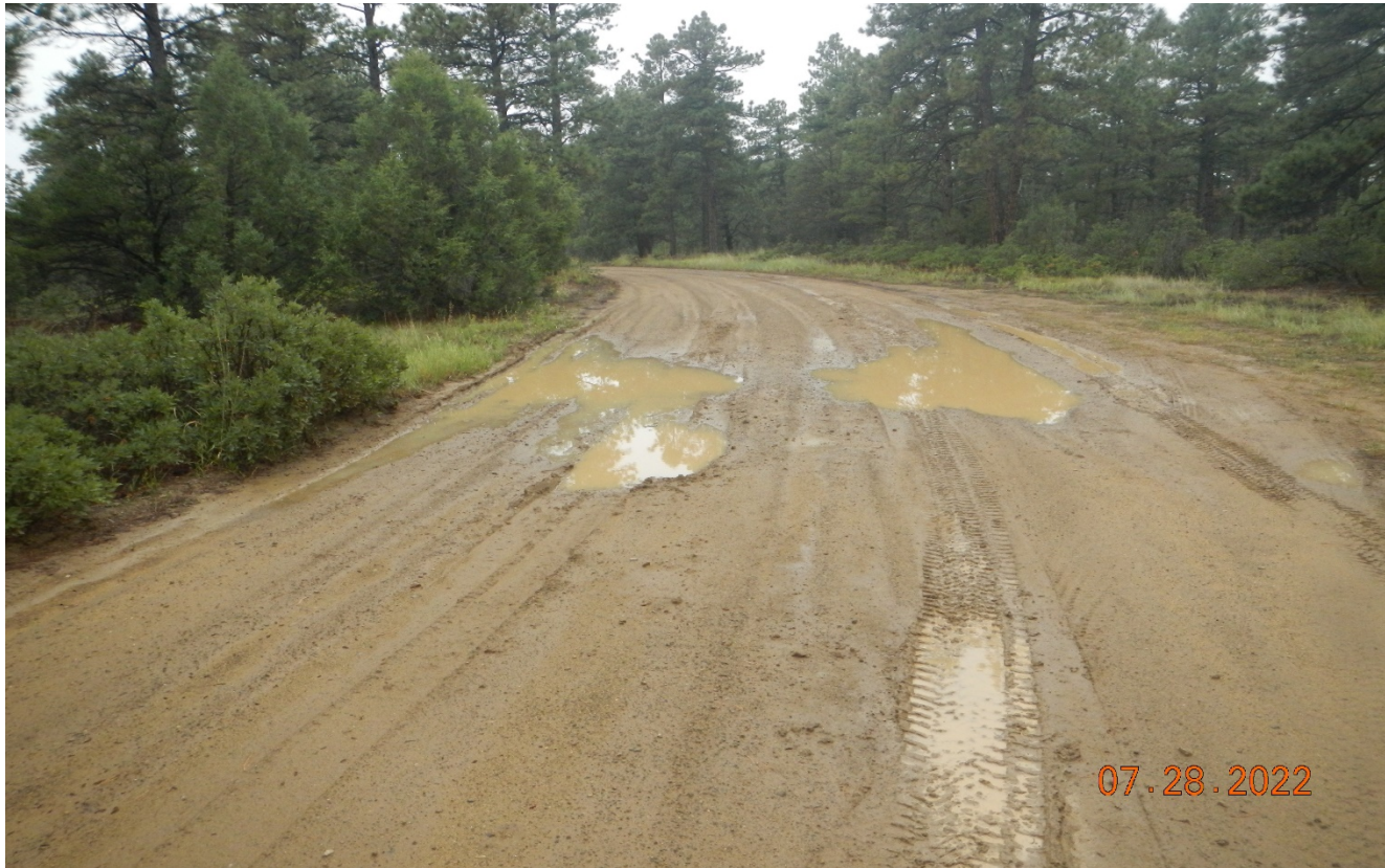
Photo 1. Facing south along the access road. There are areas where stormwater is pooling on the road causing widening of the road. This area needs additional stabilization.
