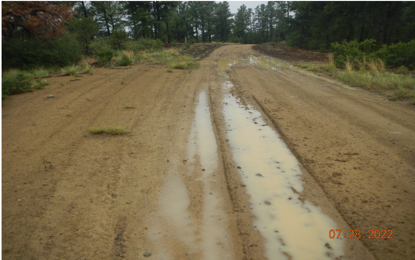
Photo 5. Facing south just past the location along the access road. There are areas where stormwater is pooling on the road causing widening of the road. This area needs additional stabilization.
