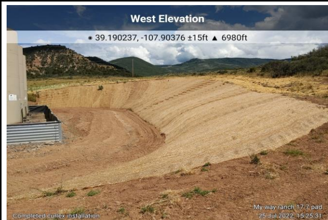
Erosion Control Blanket Installation on the MWR 17-7 Pad
