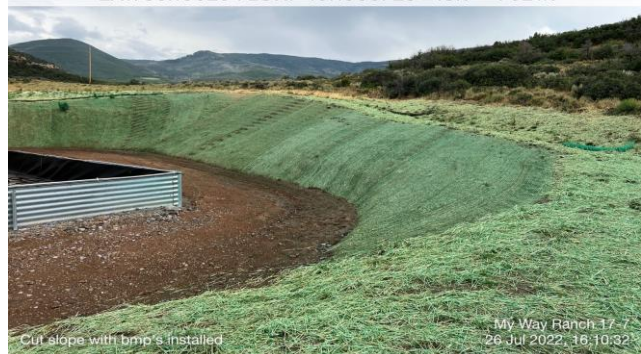
Erosion Control Blanket Installation on the MWR 17-7 Pad after Treated with Liquid Amenities
