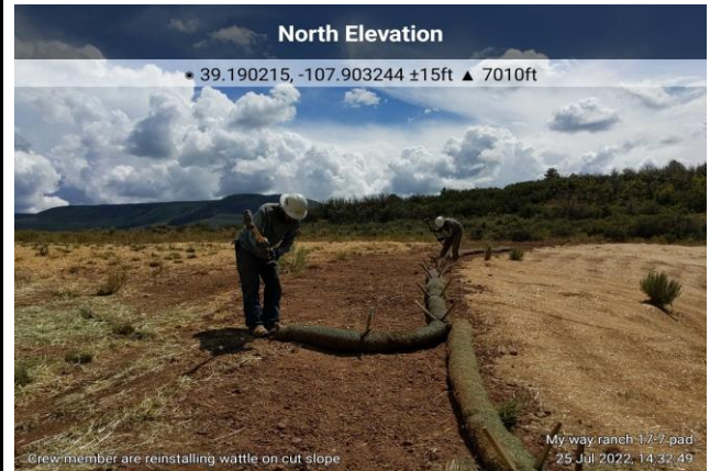
Reinstalling Excelsior Wattle on the My Way Ranch 17-7 Pad
