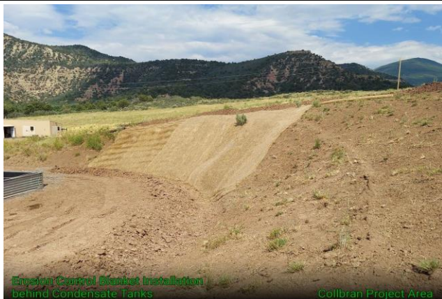
Partially Installed Erosion Control Blankets behind Condensate Tanks
