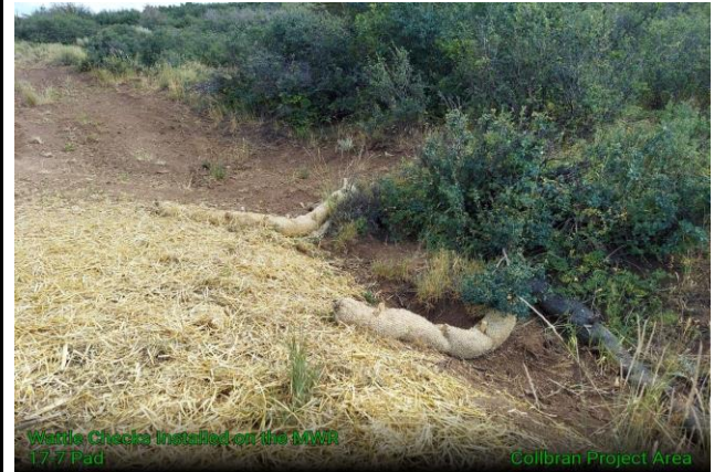
Two Wattle Checks Installed on Southwest Corner of the MWR 17-7 Pad
