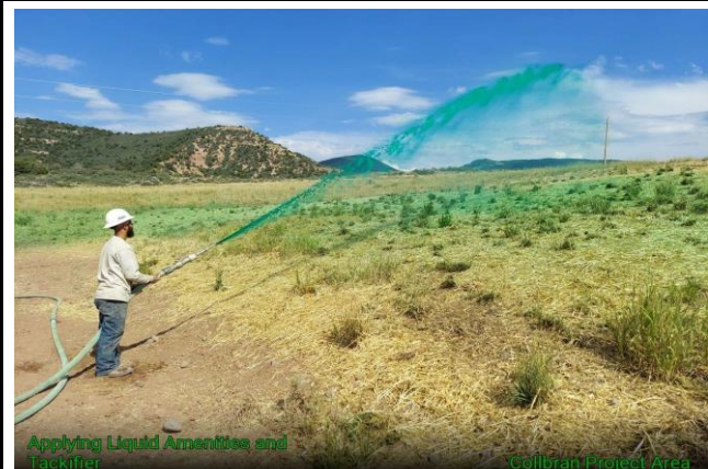
Applying Liquid Amenities and Tackifier
