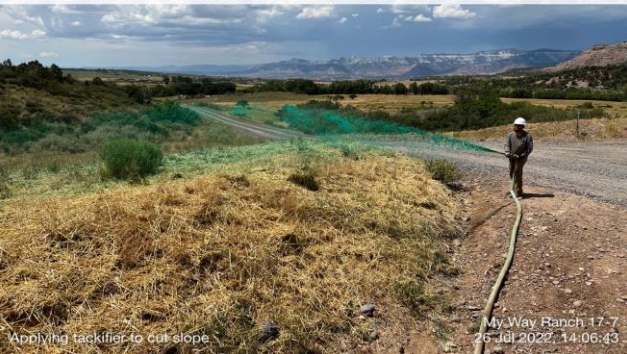
Applying Liquid Amenities and Tackifier on the My Way Ranch Pad
