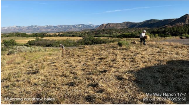
Applying Straw Mulch by Hand on the My Way Ranch 17-7 Pad
