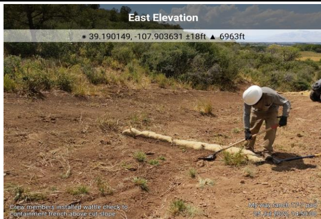
Installing New Excelsior Wattle Check
