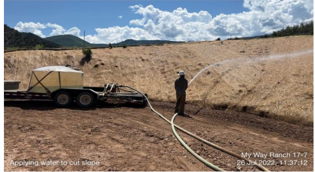
Applying Fresh Water to Erosion Control Blanket Installation
