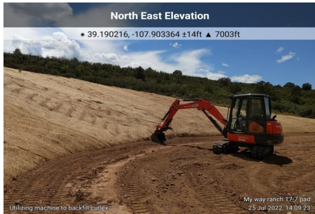
Installing Erosion Control Blanket on the MWR 17-7 Pad
