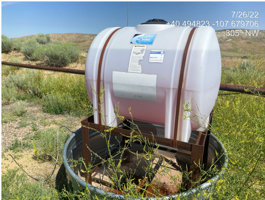
Photo 6. Photo taken from the north of the Location shows a methanol tank. The secondary containment stock tank lacks wildlife protection BMPs. Safety labeling on the tank is faded and/or peeling and inadequate.
