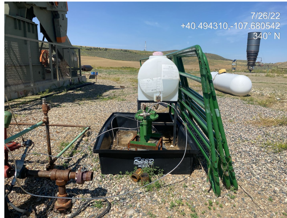
Photo 7. Photo taken from the well area shows a methanol tank lacking wildlife protection BMPs on the secondary containment device.
