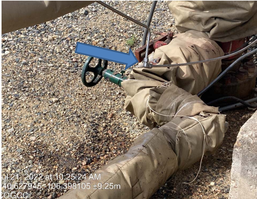
Staining and arrow is pointing at leak in chemical line
