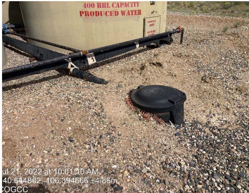
Earth berm not sufficient for a spill
