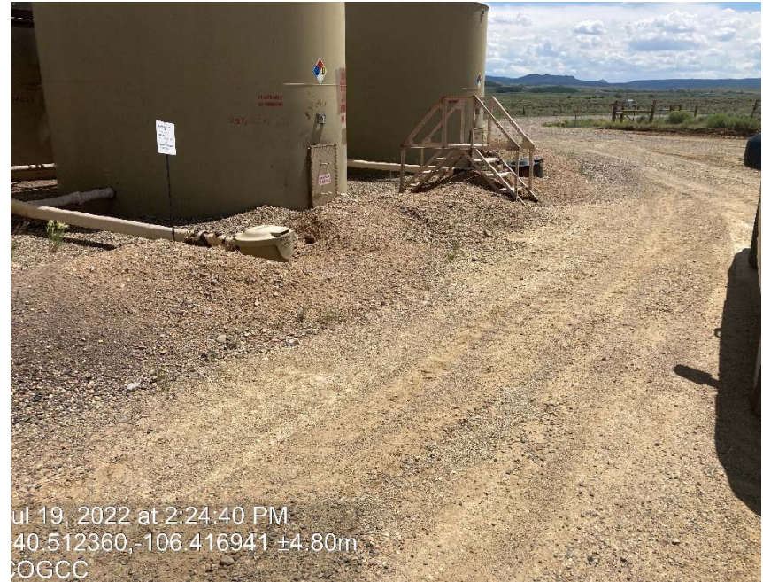
Berm dug out for load out buckets. Not adequate to contain a spill.
