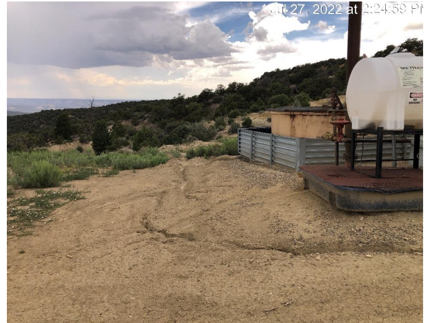
Storm water damage around tank and metershed.
