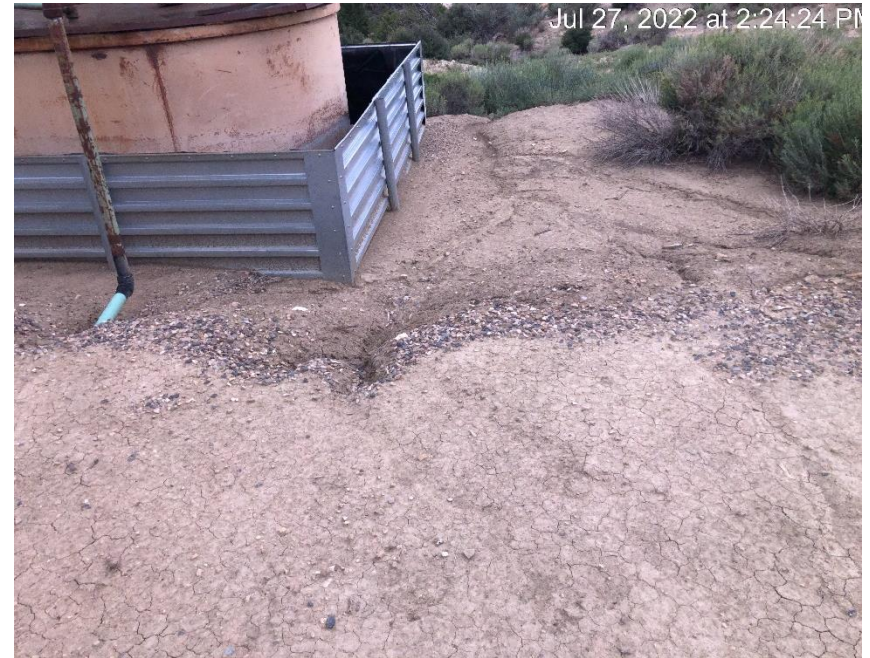
Storm water damage around tank and metershed.
