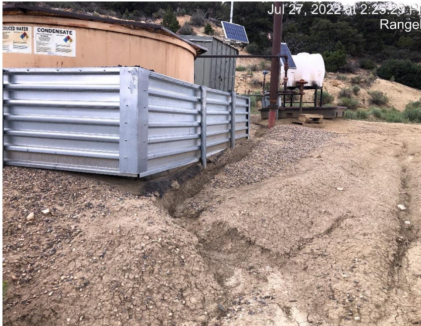
Storm water damage around tank and metershed.
