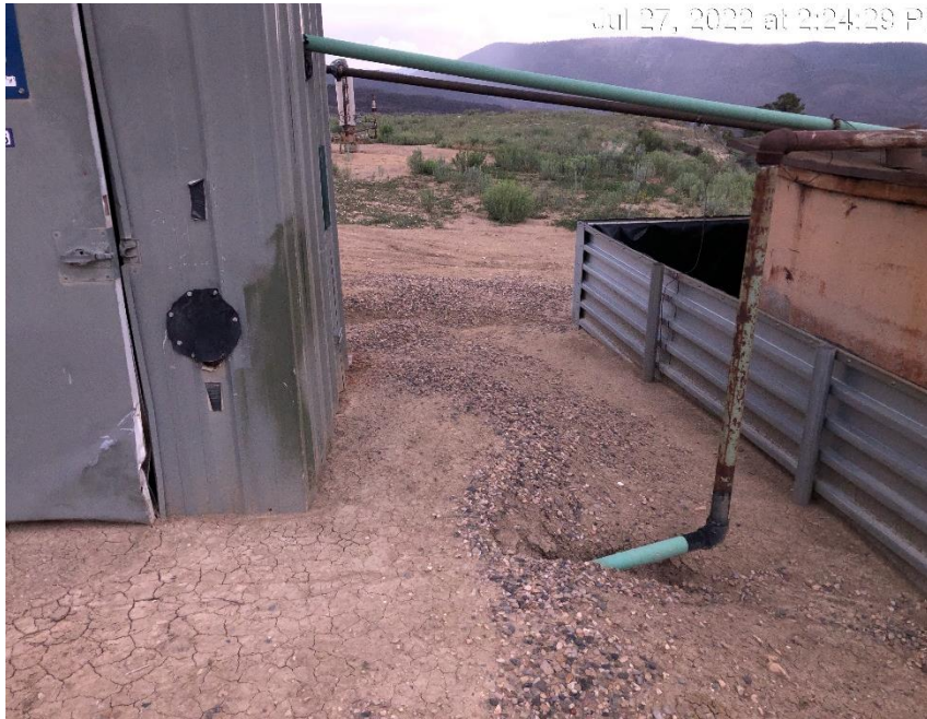
Storm water damage around tank and metershed.
