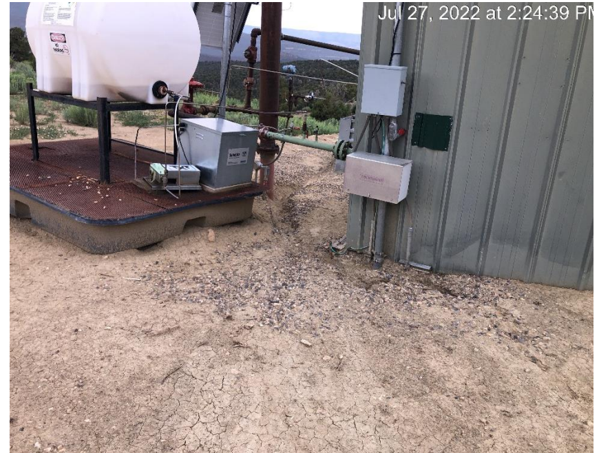
Storm water damage around tank and metershed.
