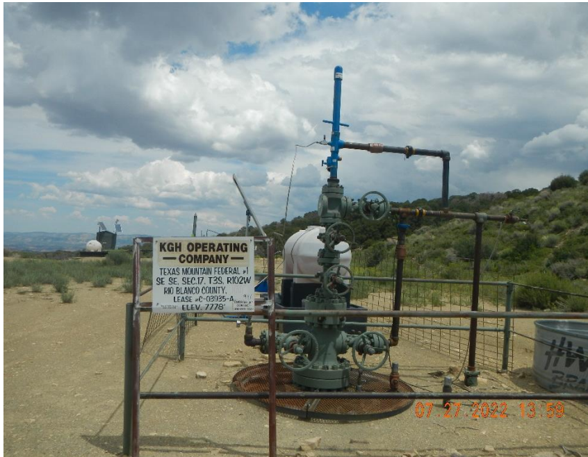
No api # on well sign.
