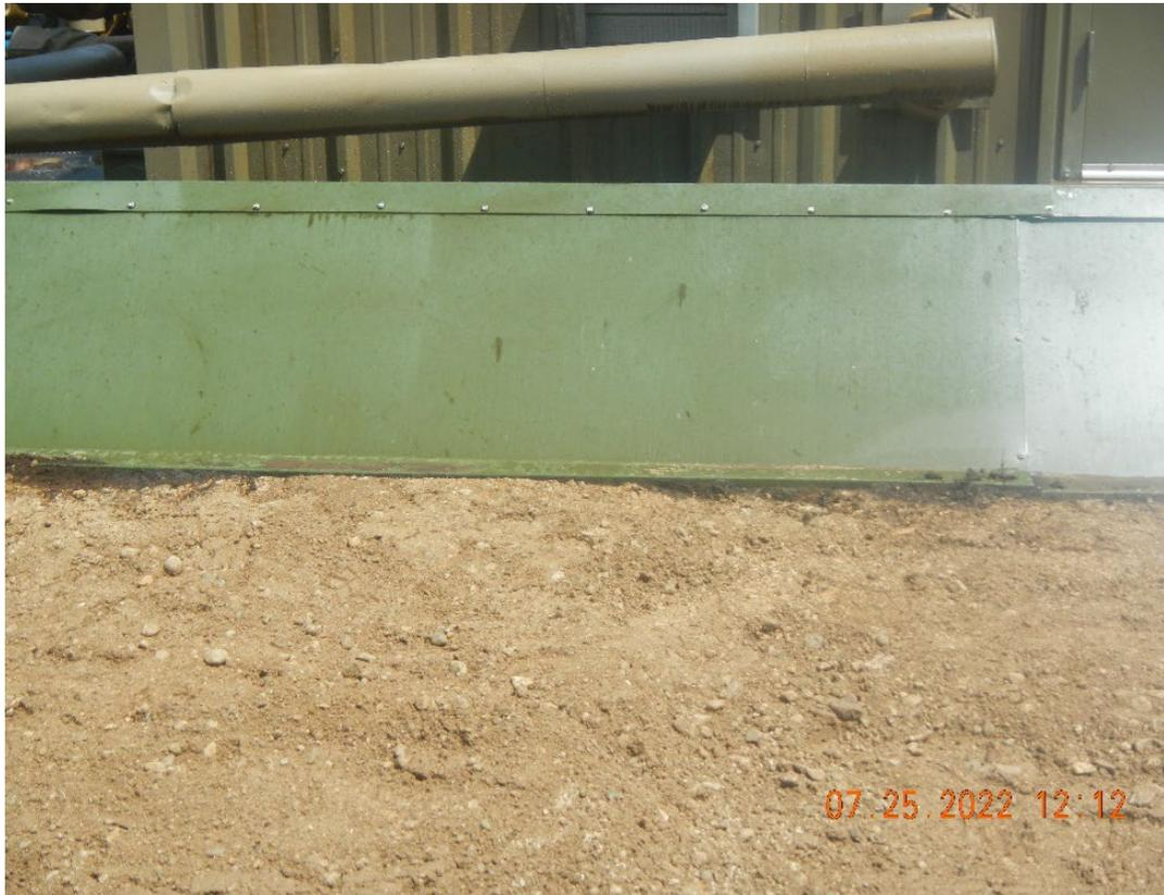
**Photo #2 photo is showing secondary containment of triplex pump, it appeared that some black staining was below the secondary containment. The source of the staining is not conclusive by observation.**
