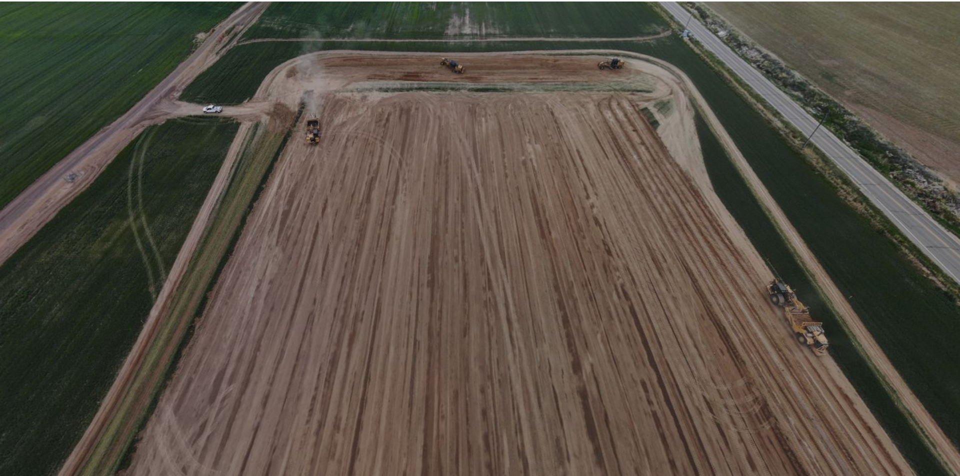
Photo 1. Drone imagery from 6/9/2022 illustrates the central-southern location during active construction operations. Topsoil has been stockpiled along the southern perimeter of location. Photo also illustrates the perimeter ditch and berm BMP.
