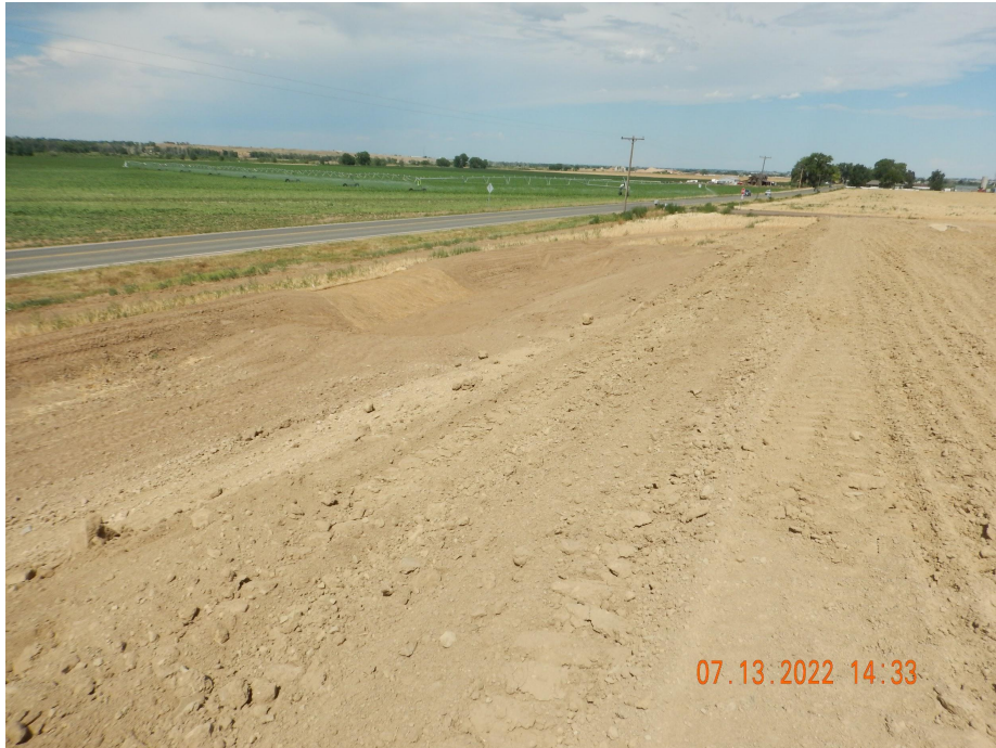
Photo 7. Photo taken from the northeastern location, facing Northeast. Photo illustrates a sediment trap BMP with a temporarily stabilized outlet.
