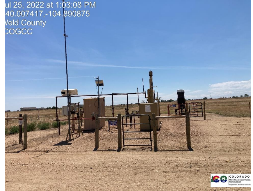
Pic 2 Gas meter run, separator, ECD
