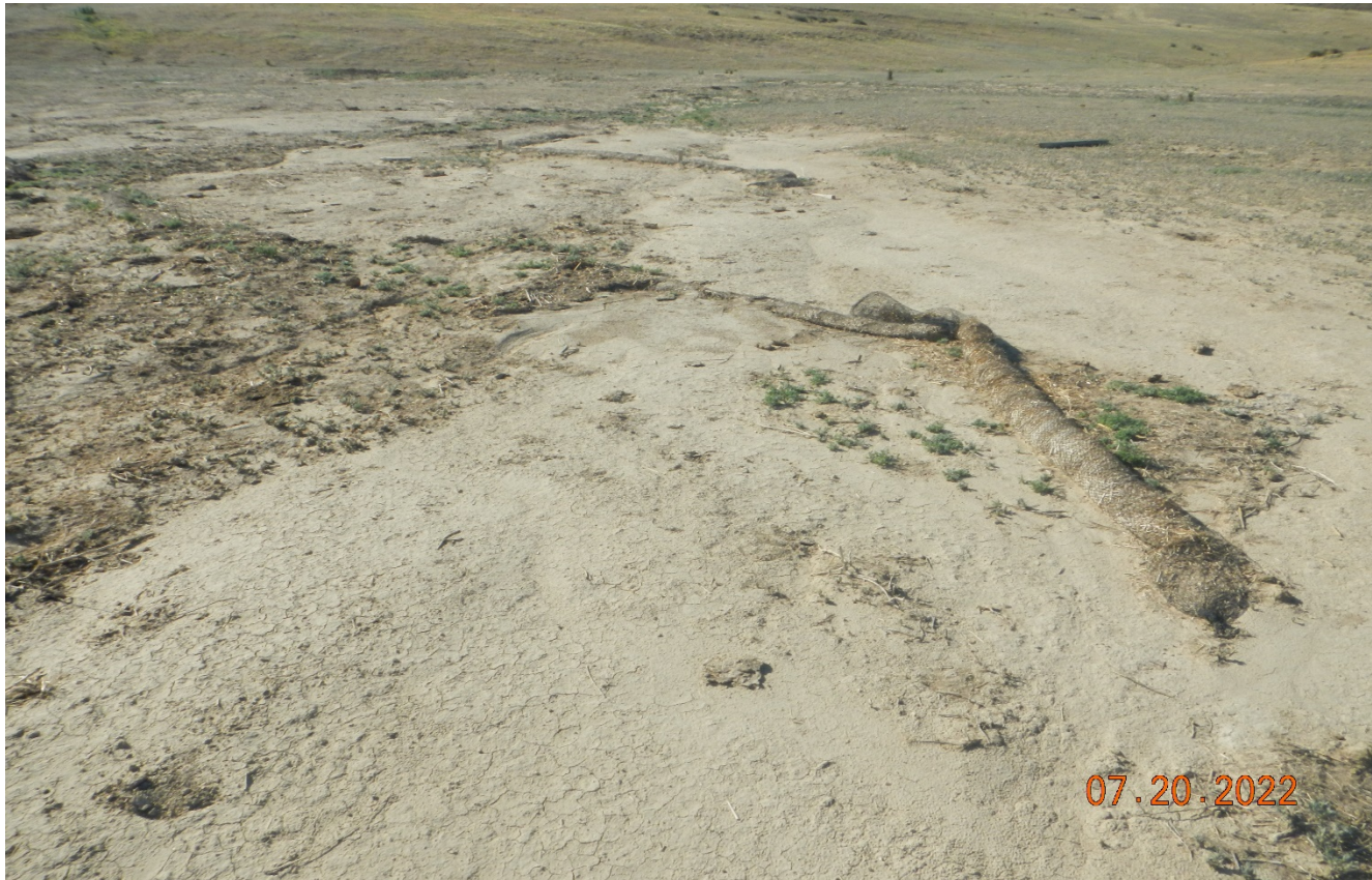
Photo 4. There are degraded and displaced wattles that are now debris. BMP's must be installed and maintained.
