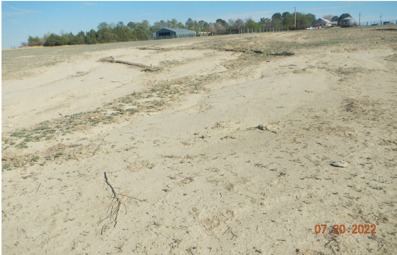
Photo 5. Facing northwest at the location. There are signs of erosion and soils are not stabilized. BMP's must be installed and maintained.
