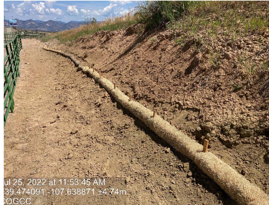
Cut slope not stabilized
