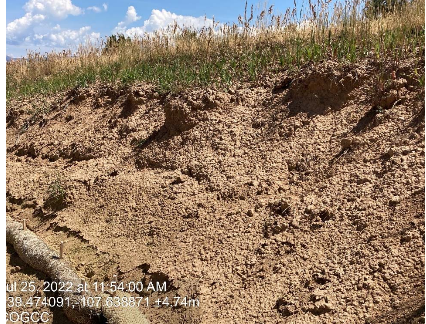
Cut slope not stabilized
