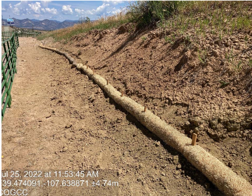
Cut slope not stabilized
