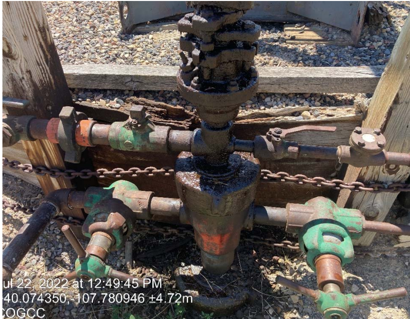
Leaking stuffing box
