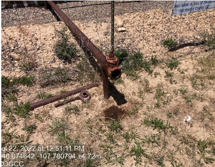
Staining and lacking cap/bull plug
