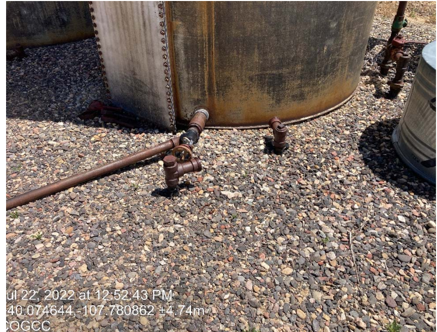
Lines form tanks to unlined pit
