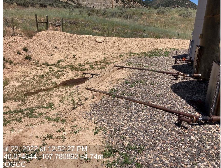
Lines form tanks to unlined pit
