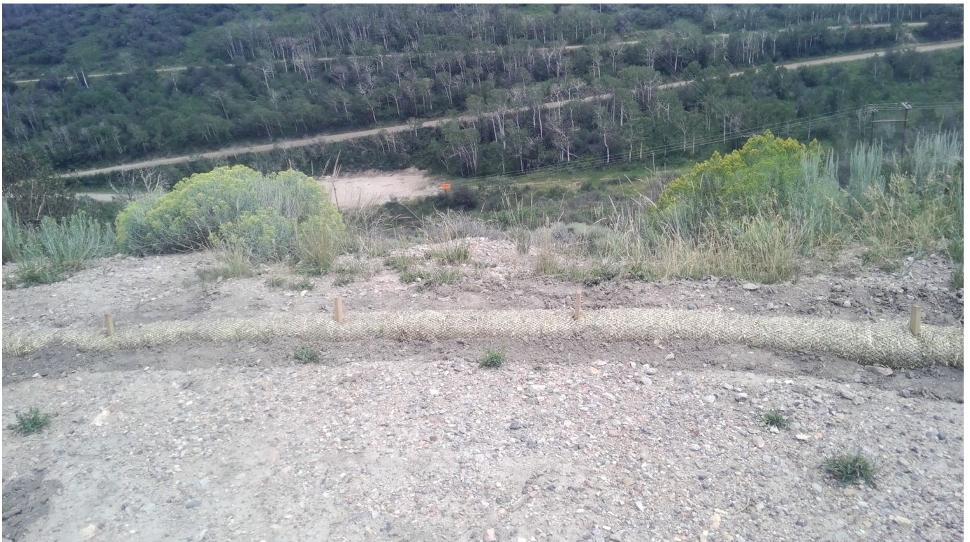
CA2: Debris has been removed & CA4: BMP's installed
