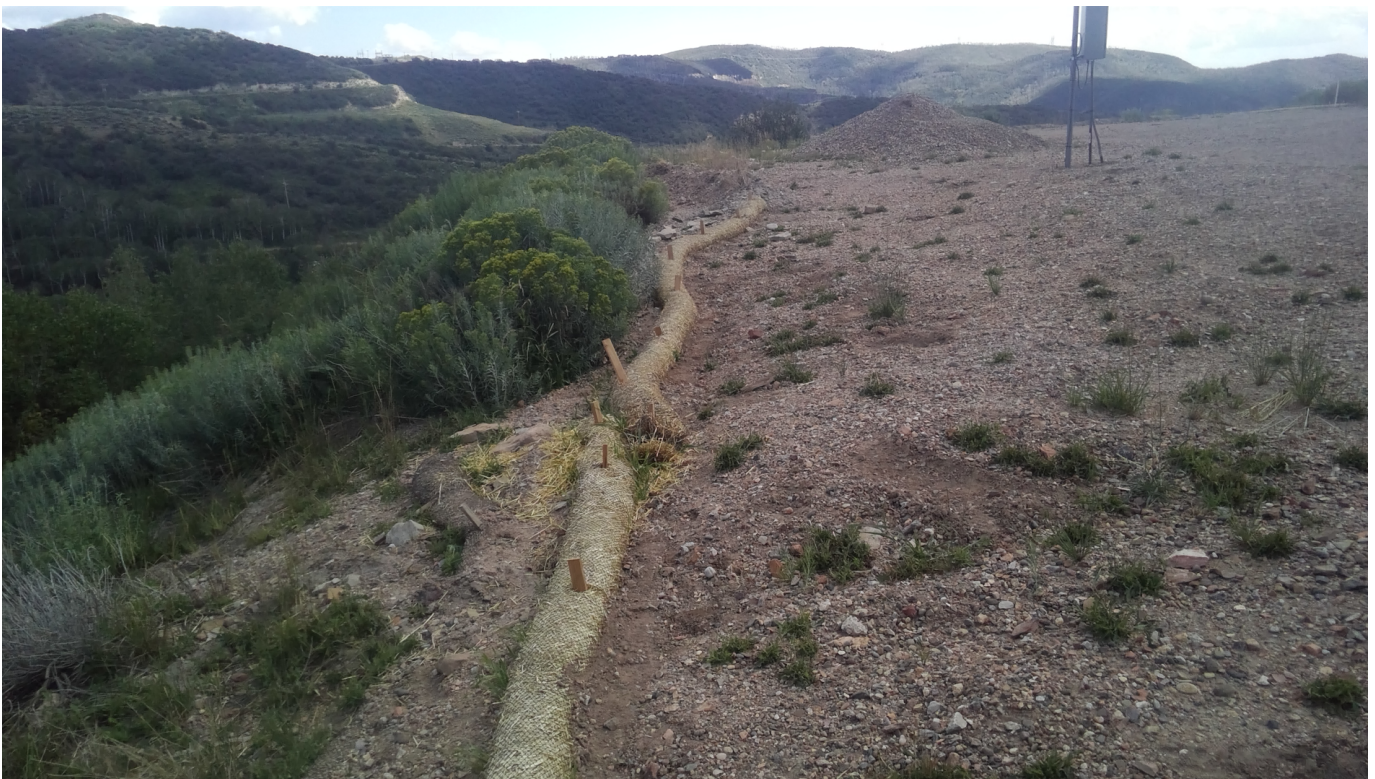
CA4: BMP's installed
